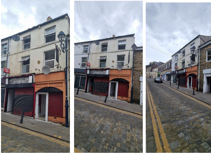
Figure 2: Existing principal elevation viewed from Daisy Hill showing the existing white rendered facade, roller shutters, entrance doors and the current condition of the building.
