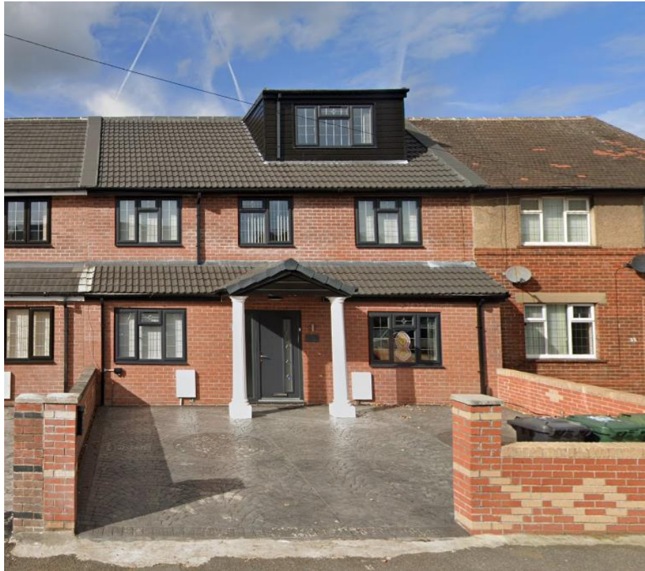
5.14 Above: Similar size and design of dormer at 20 Lee Road opposite.
