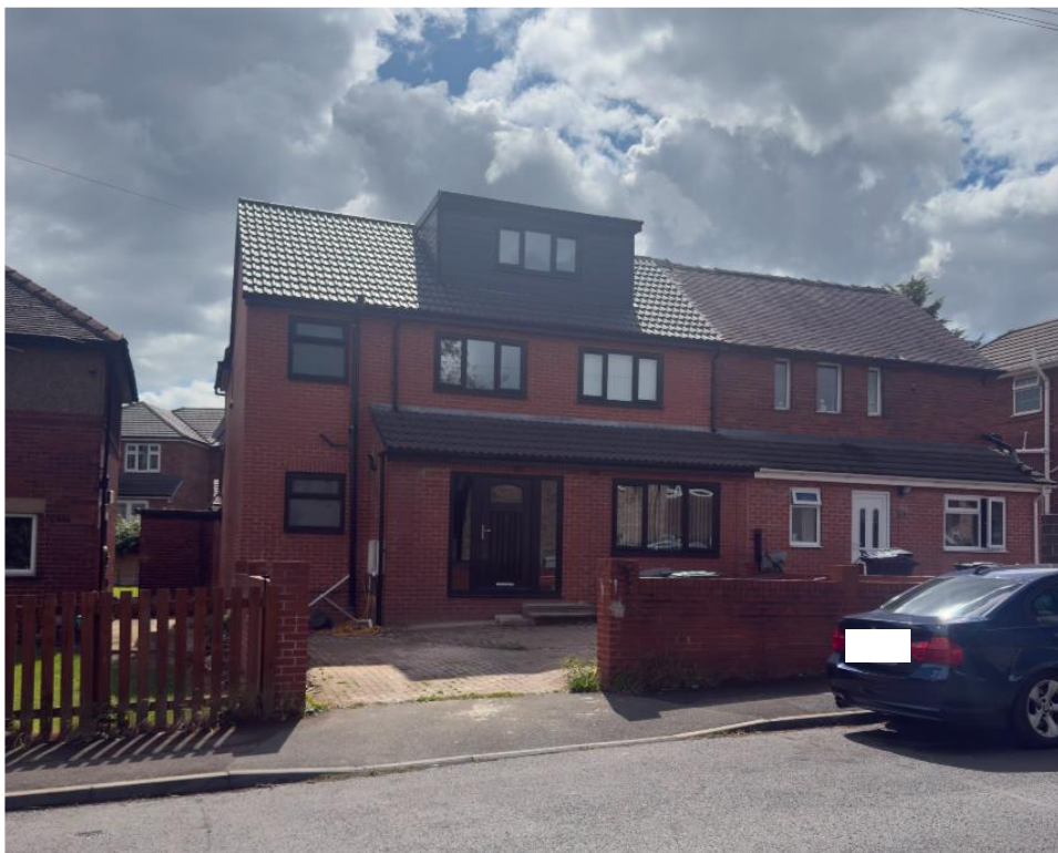
5.15 Above: Similar size and design of dormer at 94 The crescent.
