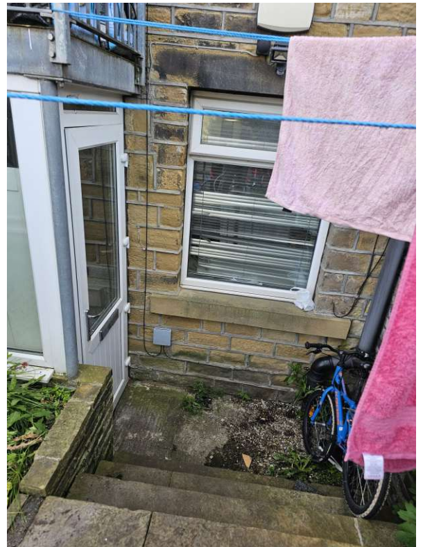
ENTRANCE TO BASEMENT
