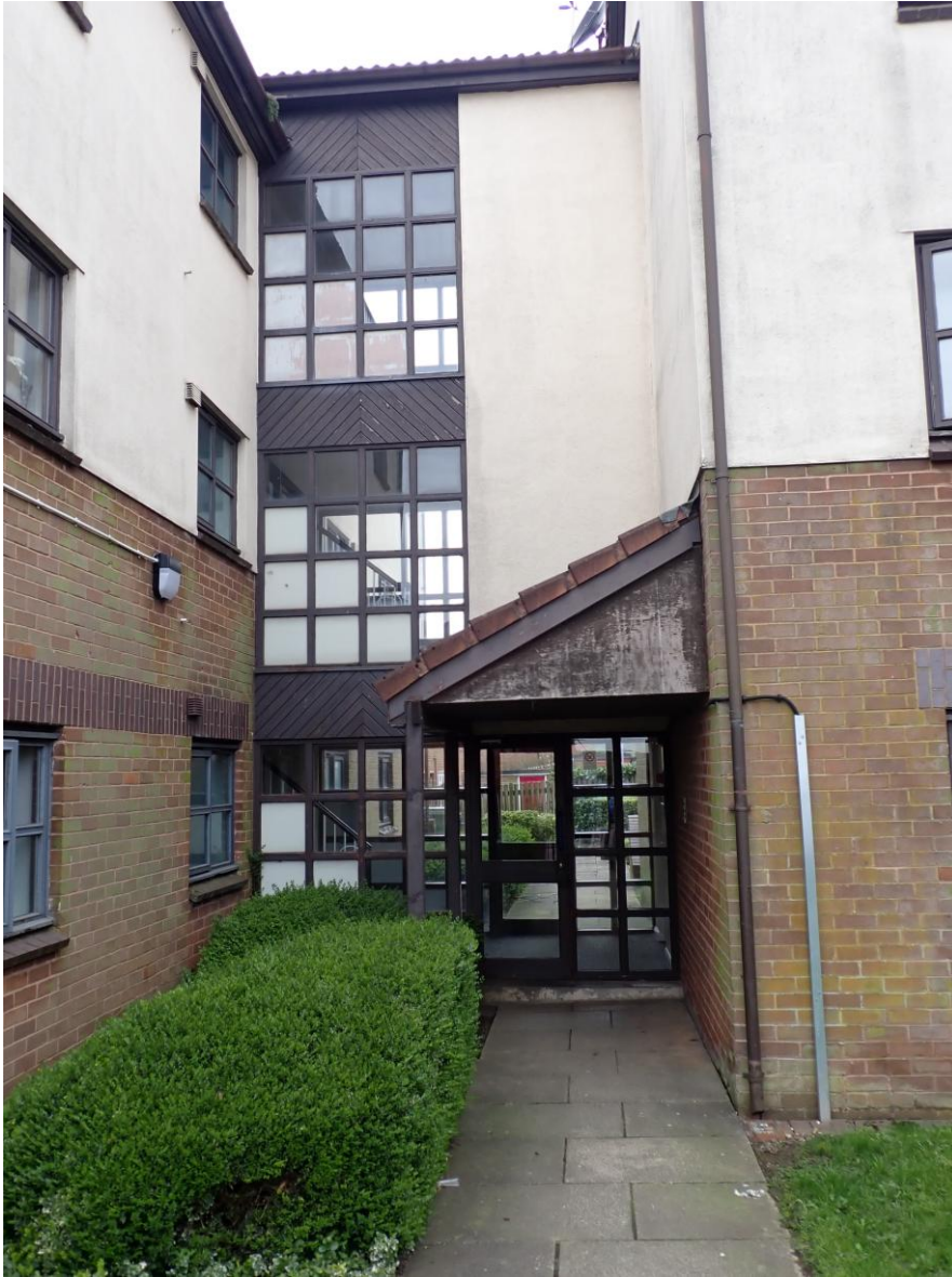
Photograph 1—Typical Curtain Walling
