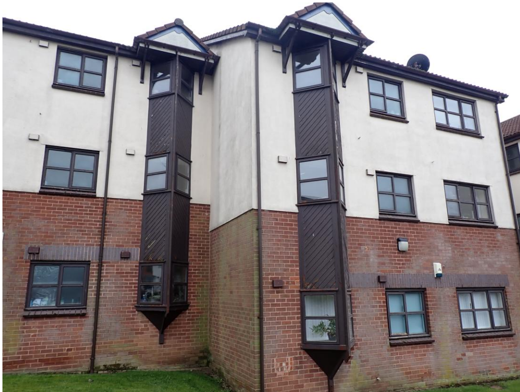
Photograph 2—Typical Windows, Timber Bays and Roof Gable
