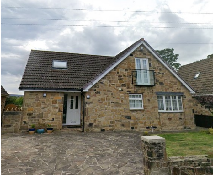
Figure 2: 115 Caldercliffe Road — two storey garage attachment with front entrance door, matching stone throughout.
