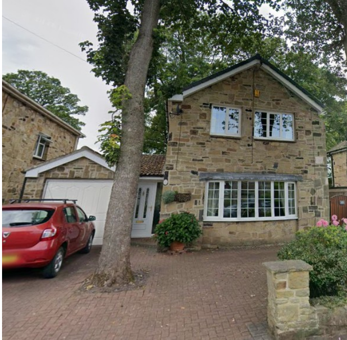
Figure 4: 121 Caldercliffe Road — single storey garage attachment with front entrance door, and two storey rear extension.
