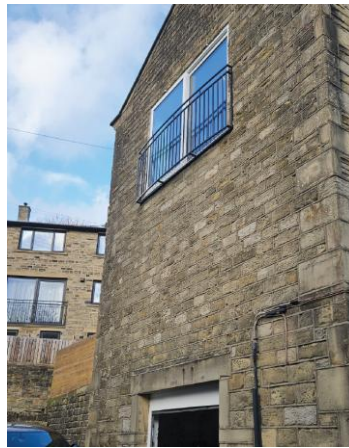
Figure 1: The existing Juliet balcony in the foreground with the similar designed Juliet and balustrade to 119A Woodhead Road in the background
