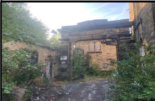
Photograph 3. The entrance of the Site
