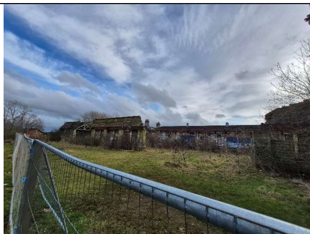
Photo 10: built linear features and mixed scrub at the south of the site.
