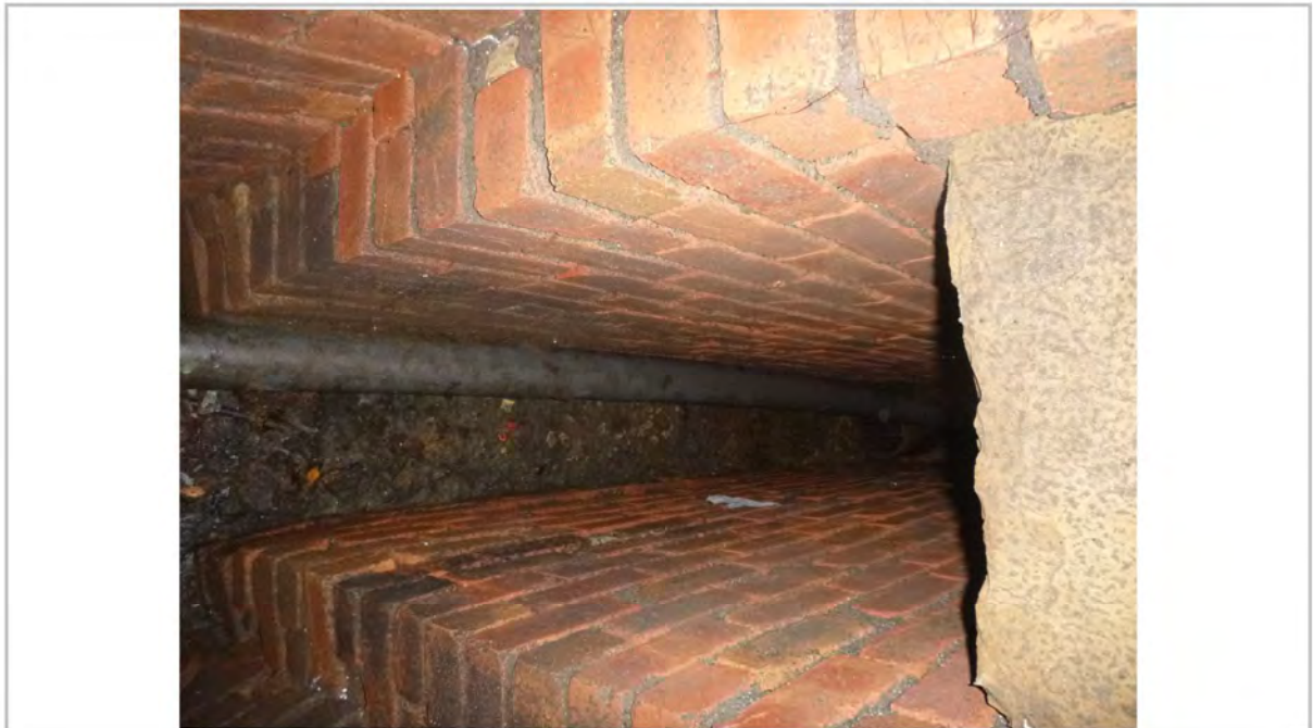
GP23 EDS3 - VIEW UP DUCT FROM CHAMBER
