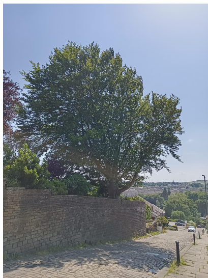
T1 + Boundary Wall
