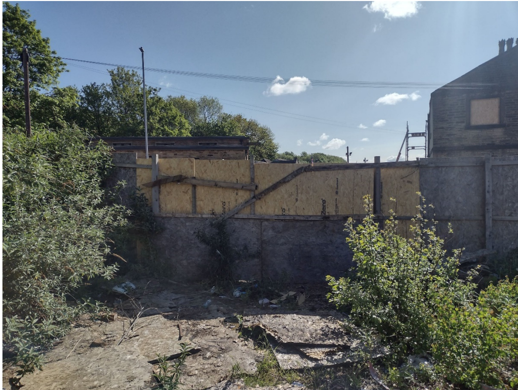
Photograph 1: Boarding along former access off Dowker Street along the eastern boundary of the site.
