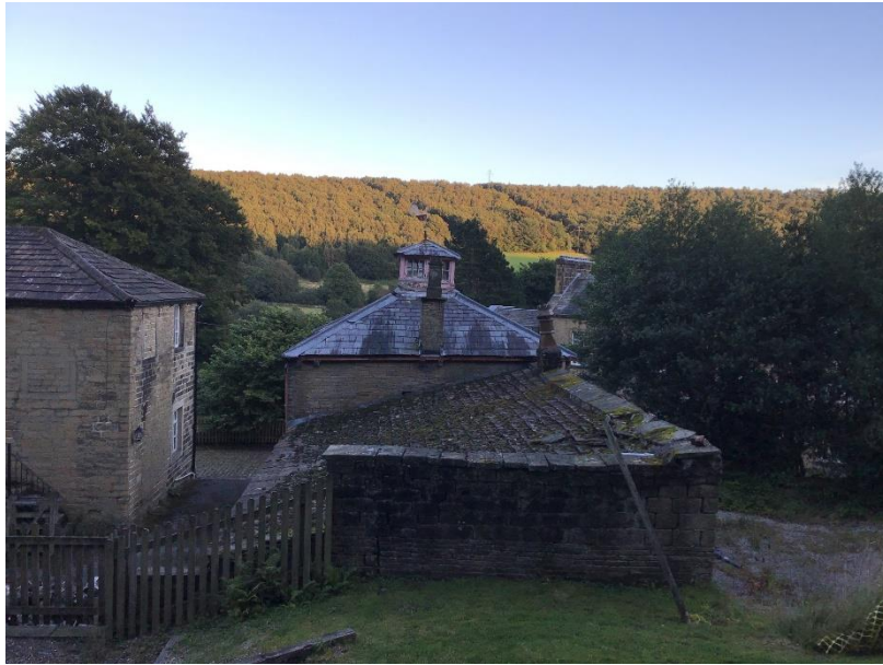
North aspect, with extension in foreground
