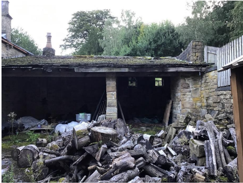
Extension, east aspect
