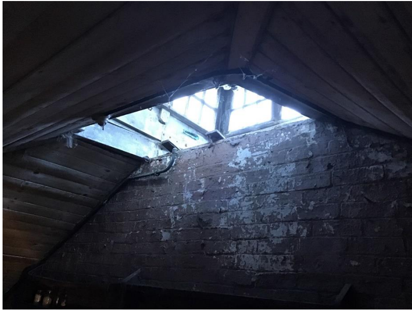
Skylight and sarking
