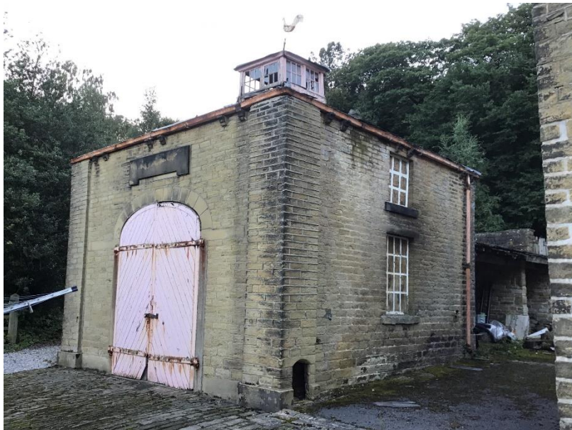
South and east aspects
