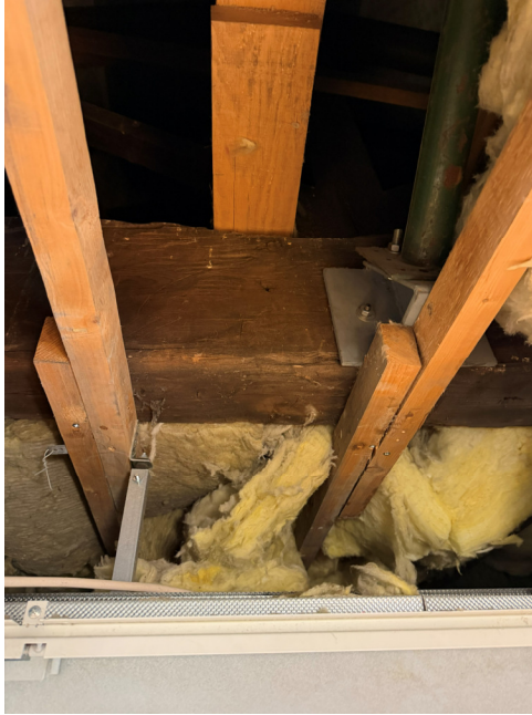
Figure 3 – Image looking through the loft hatch to the underside of the existing roof structure. The historic truss in dark wood and lighter wood being more recent interventions. Note the suspended ceiling system hangers and loft insulation packed between the joists.
