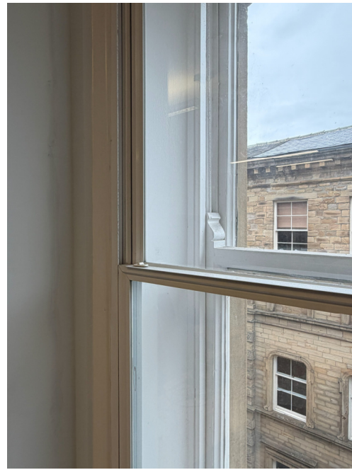
Figure 4 -Existing secondary glazing demonstrating the slimline frame profile and its discreet relationship with the historic window fabric.
