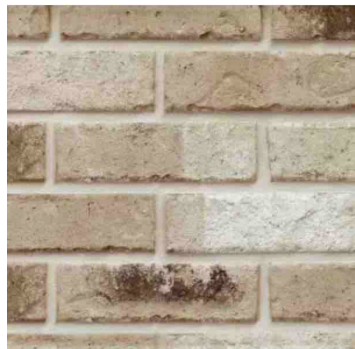
External Walling – Buff Brickwork – Cream mortar.
