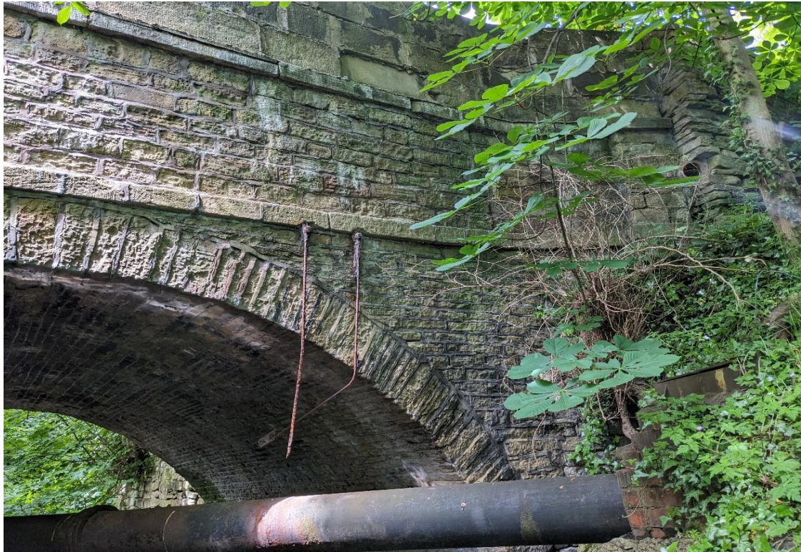
Photograph 16 - General View Of South East Spandrel Wall
