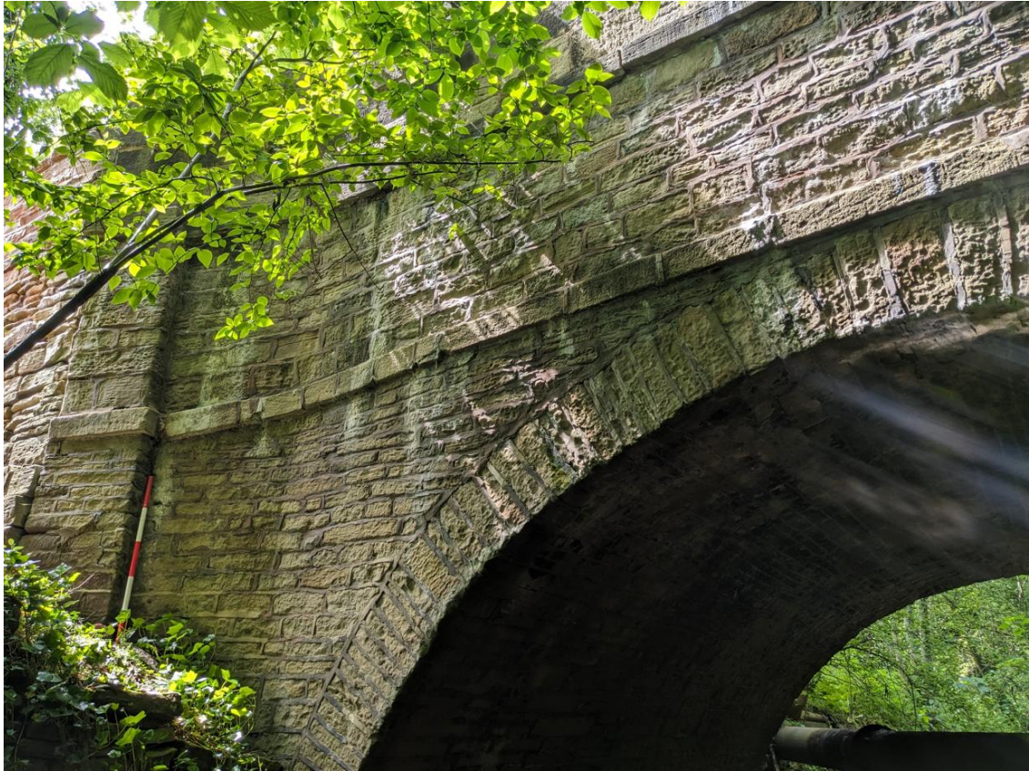
Photograph 15 - General View Of South West Spandrel Wall
