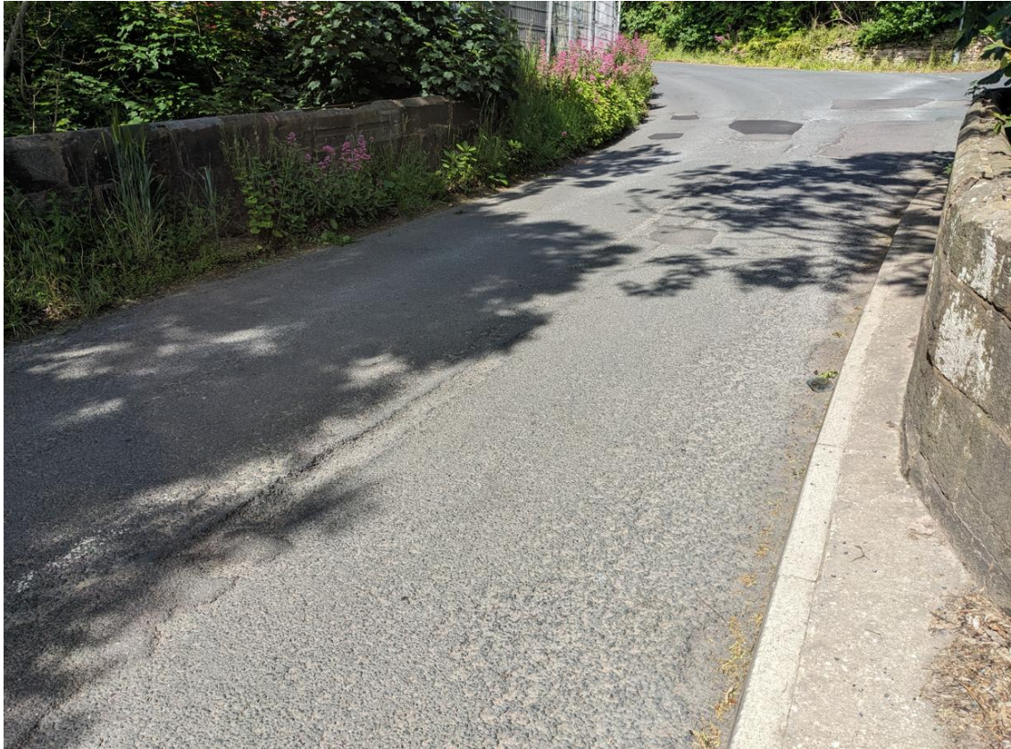
Photograph 27 - Potholing To Carriageway Surface Now Repaired
