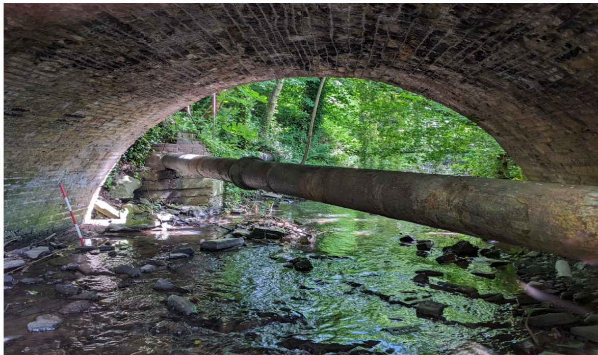
Photograph 4 - General View of Invert
