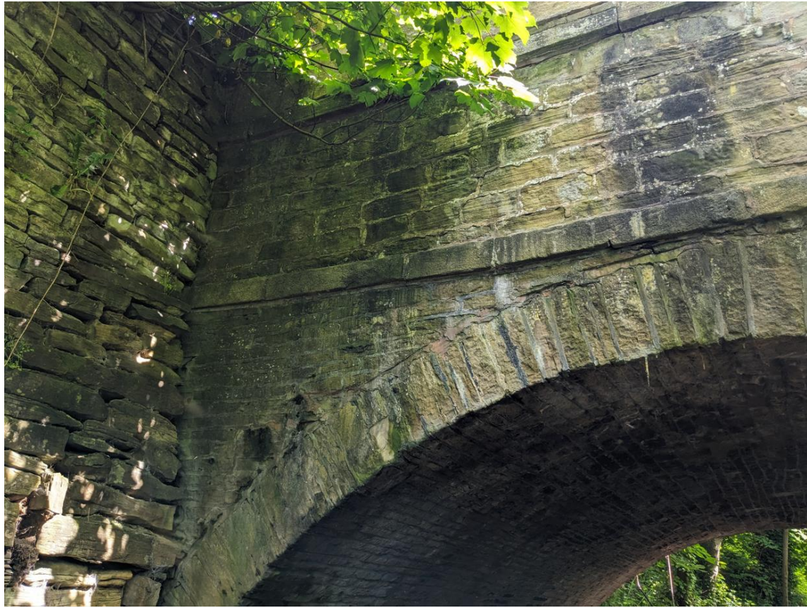
Photograph 17 - General View Of North East Spandrel Wall
