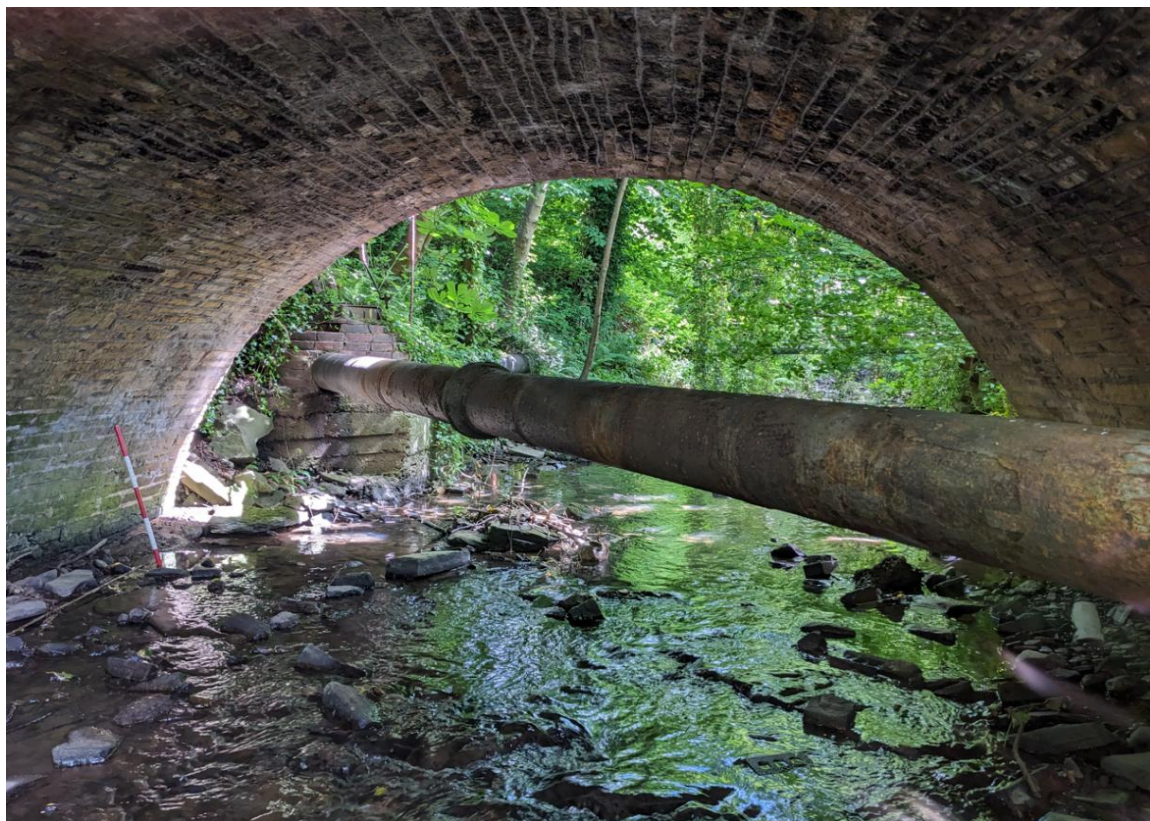
Photograph 8 - Service Pipe Running Beneath Structure
