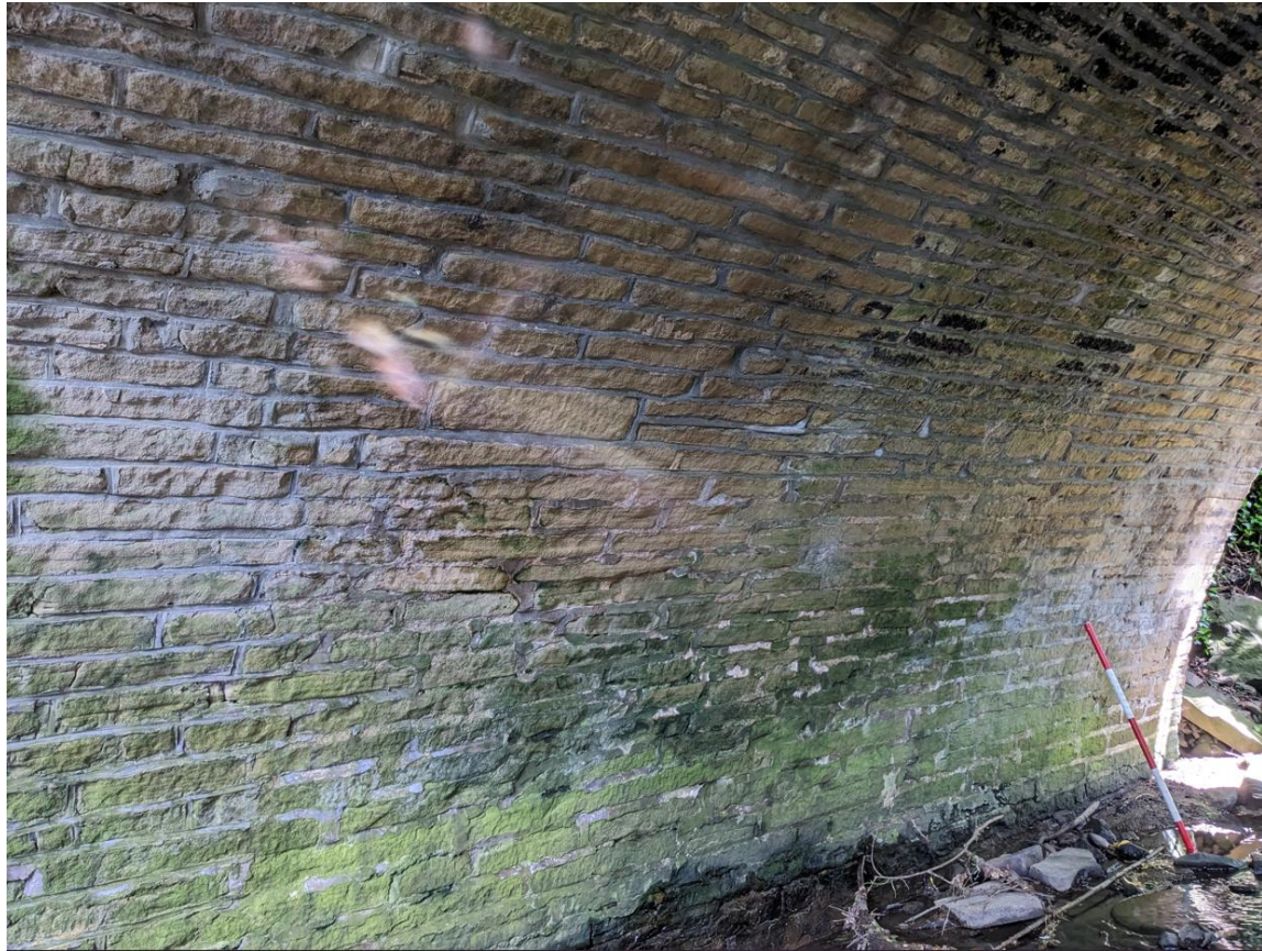
Photograph 9 - Repointing To Arch Barrel Sound
