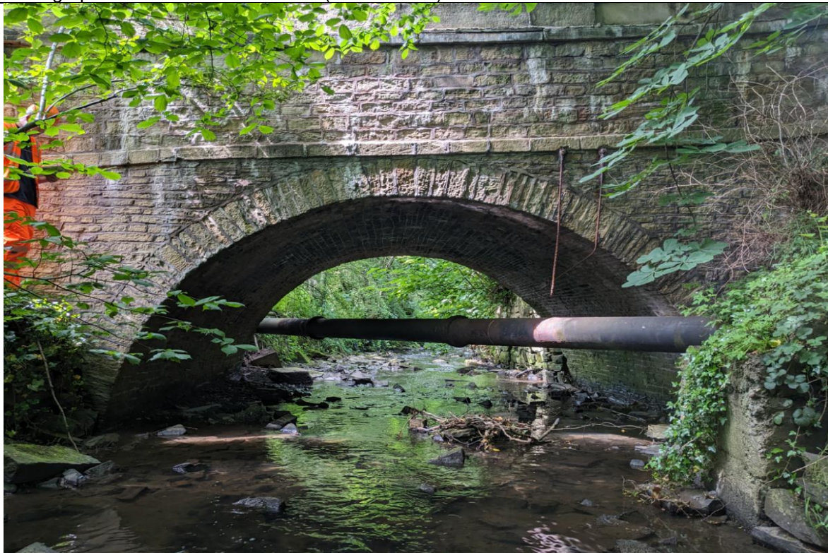
Photograph 2 - General View of South (Upstream) Elevation
