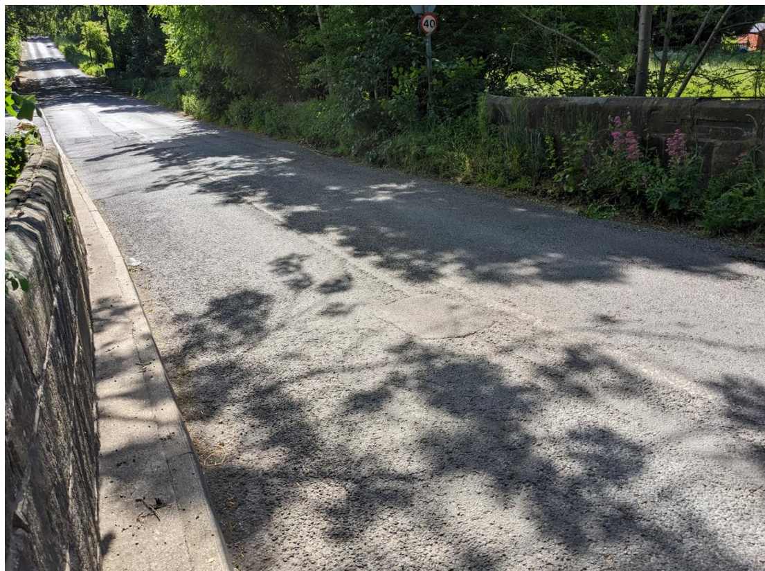
Photograph 28 - General View Over Carriageway Surface Showing Repair To Potholing
