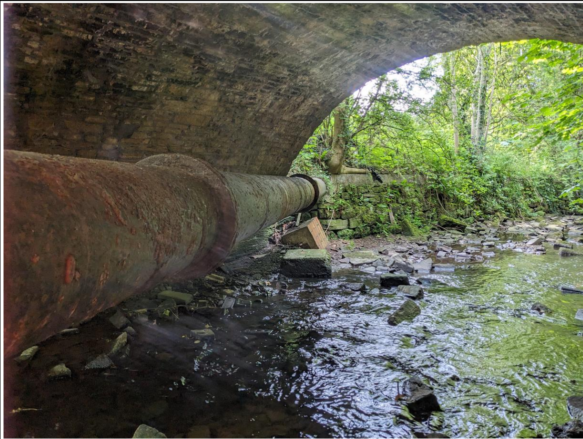
Photograph 7 - Service Pipe Running Beneath Structure
