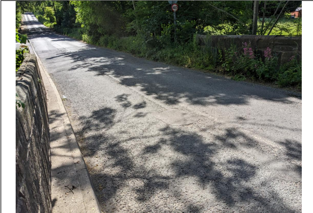
Photo C: General View Over Topside Carriageway
