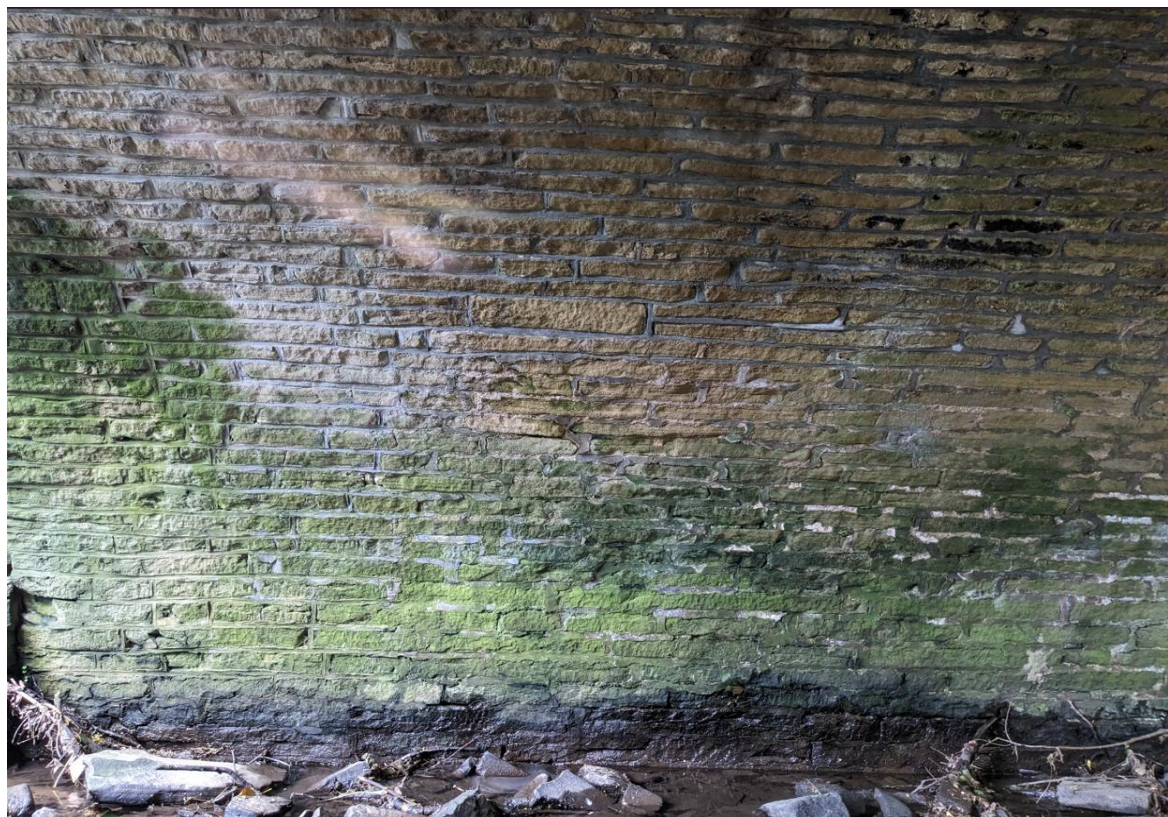
Photograph 12 - Masonry Repairs Remain Sound
