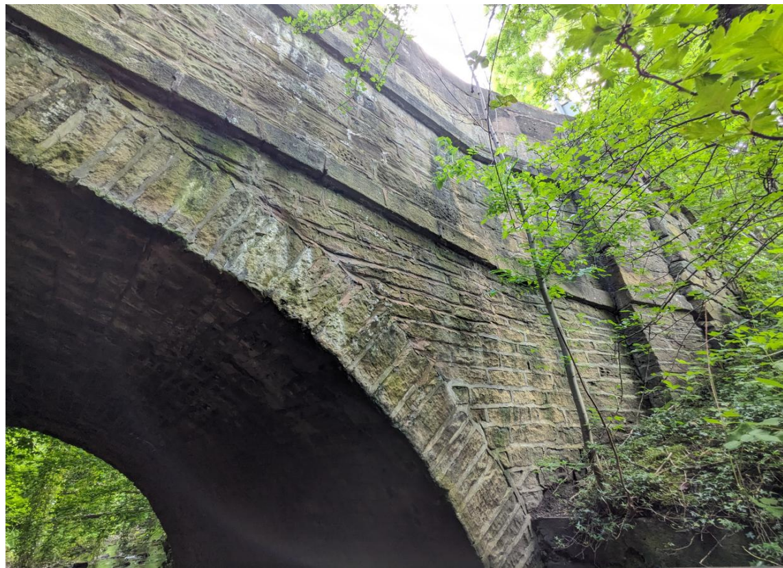
Photograph 18 - General View Of North West Spandrel Wall
