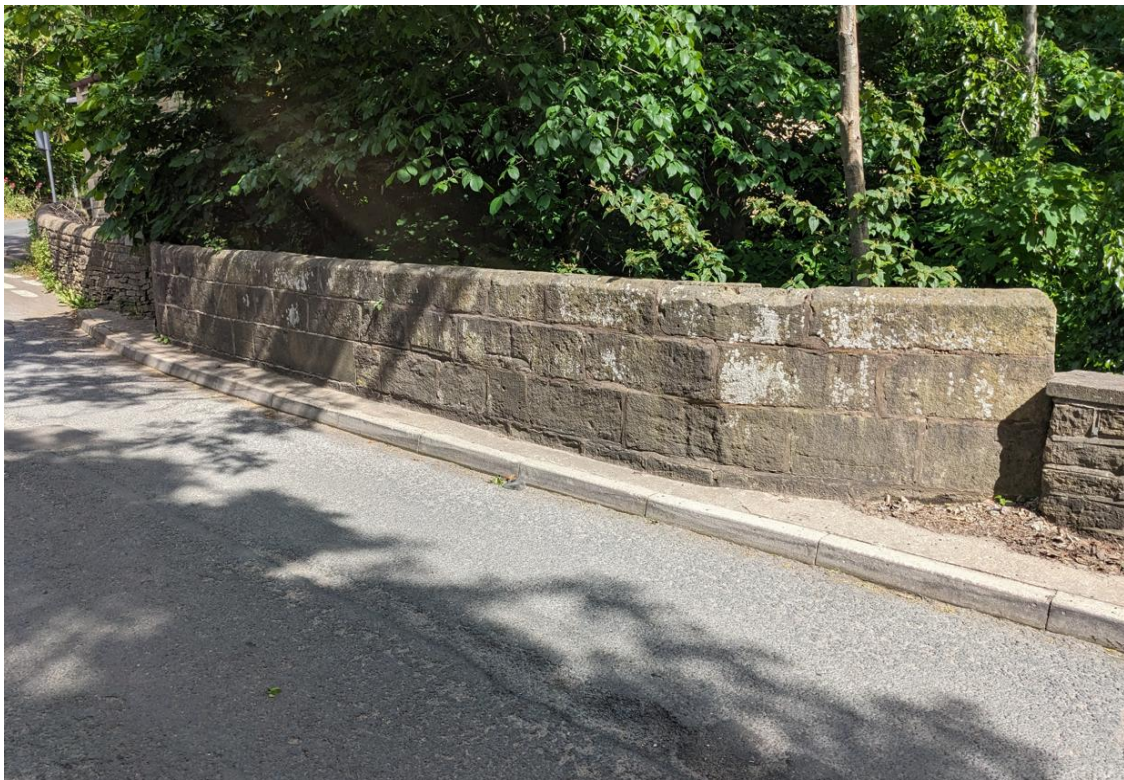
Photograph 26 - General View Along South Parapet And Verge
