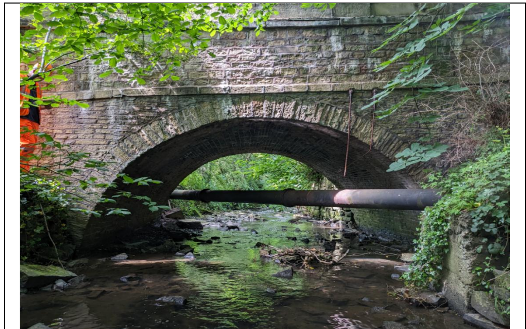
Photo B: General View of South (Upstream) Elevation
