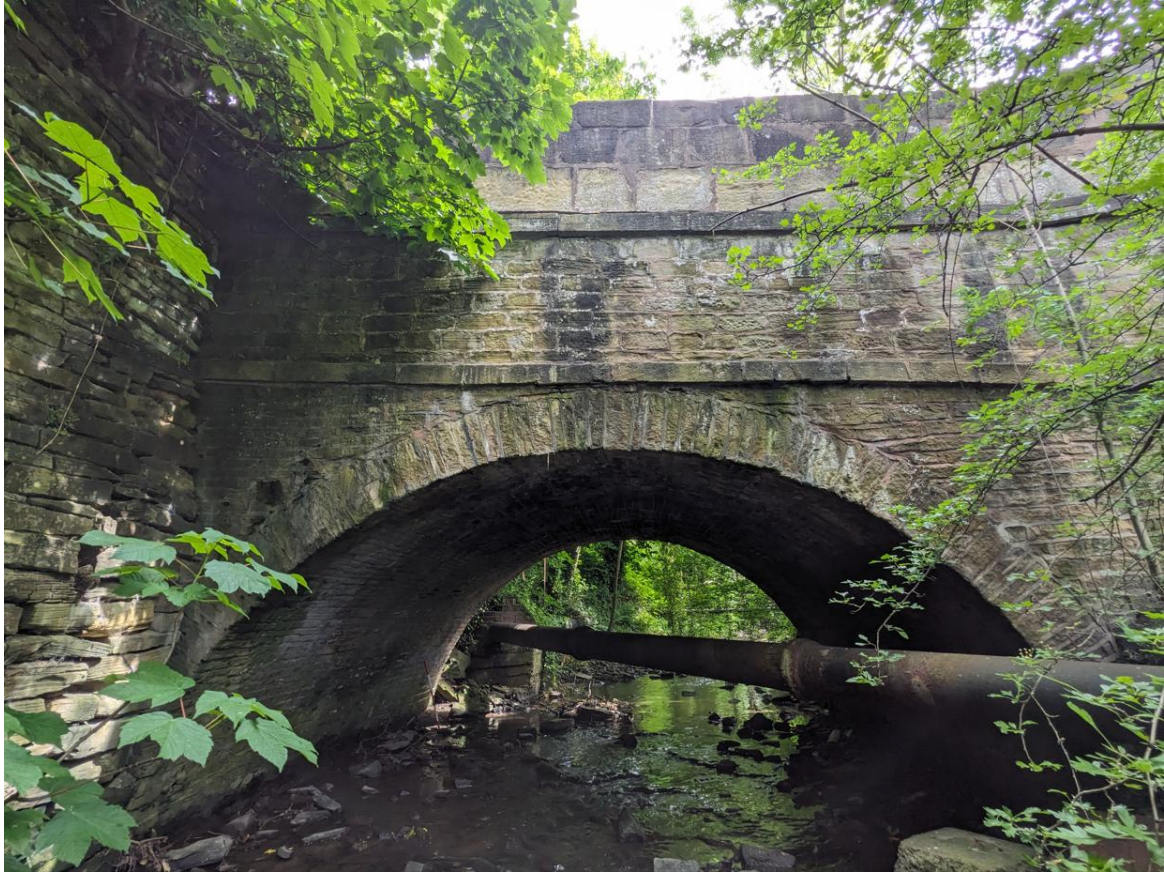
Photograph 1 - General View of North (Downstream) Elevation
