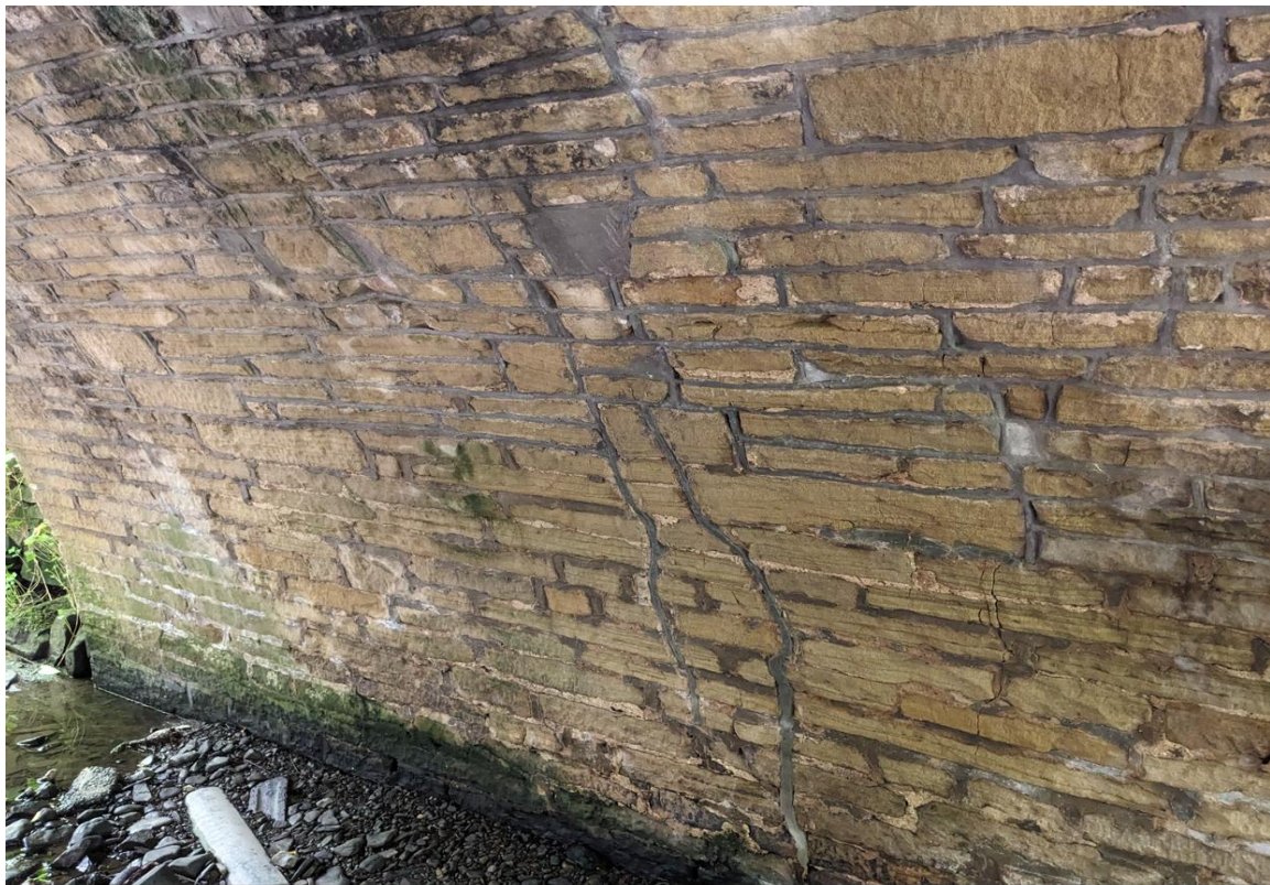
Photograph 10 - Structure Was Recently Repointed, Pointing Remains Sound
