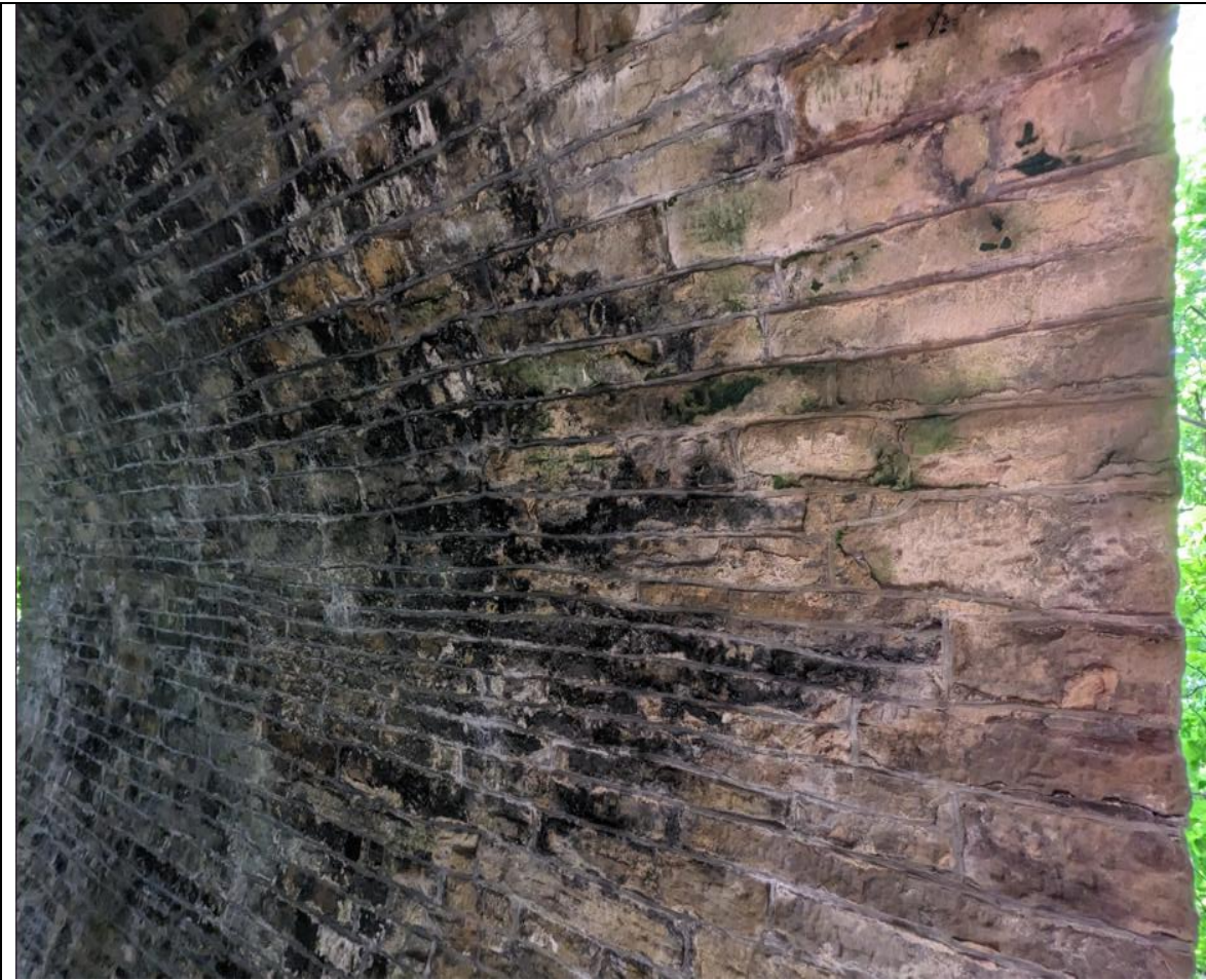
Photograph 3 - General View of Arch Barrel
