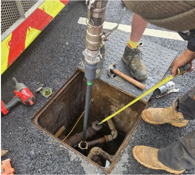
Photograph Three and Four: Pumping of residual fuel/ water mix from tanks
