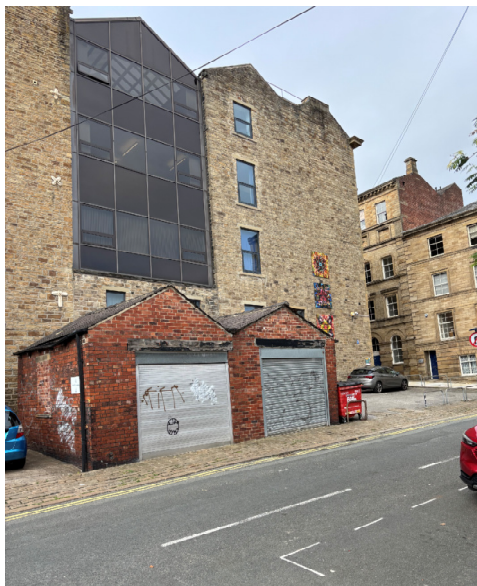
Figure 7— View of 21 Bond Street from Grove Stret. Note the artwork of 2023 to the right of the elevation.
