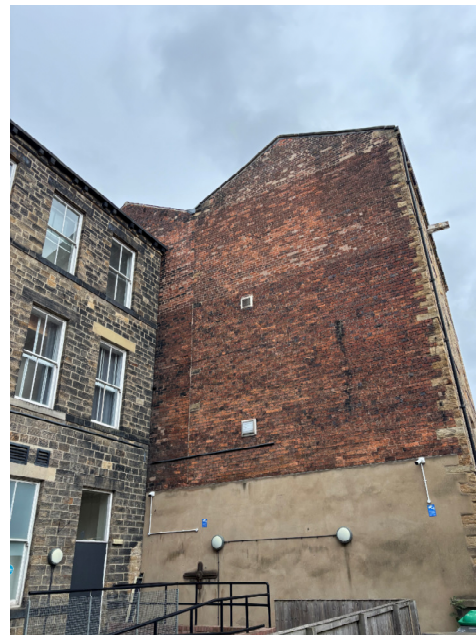
Figure 8- The west gable of 21 Bond Street
