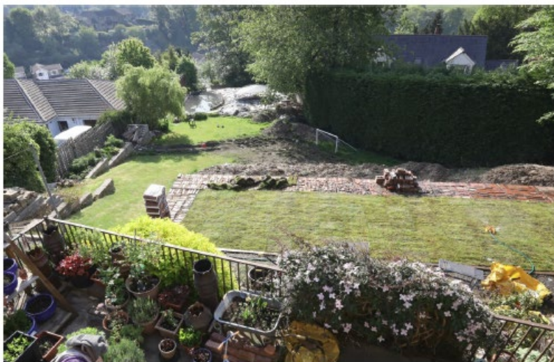
11.05.2025 – newly laid turf on the completed terrace above.
