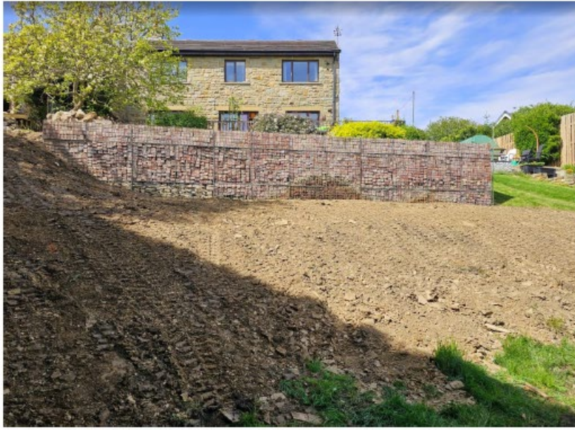
Photos after the ground has been levelled back to the original sloping garden
