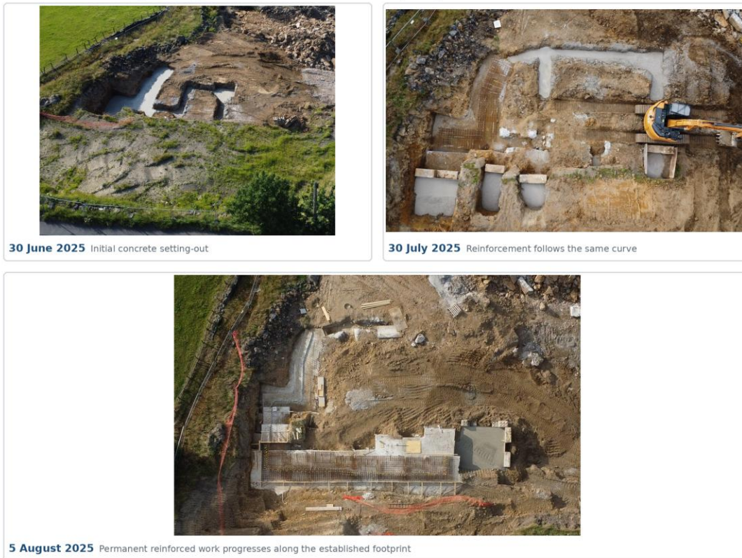
Figure 9. Dated construction sequence. On 30 June the initial concrete setting-out already defines the curved outer formation and internal foundation arrangement. By 30 July reinforcement follows the same curve and connects it into the wider layout. By 5 August permanent reinforced construction has progressed along that established footprint. The additional lower-ground geometry was therefore fixed during the original substructure works.
