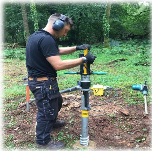
Figure 2 – Example of a hand-driven screw pile installed within an RPA
