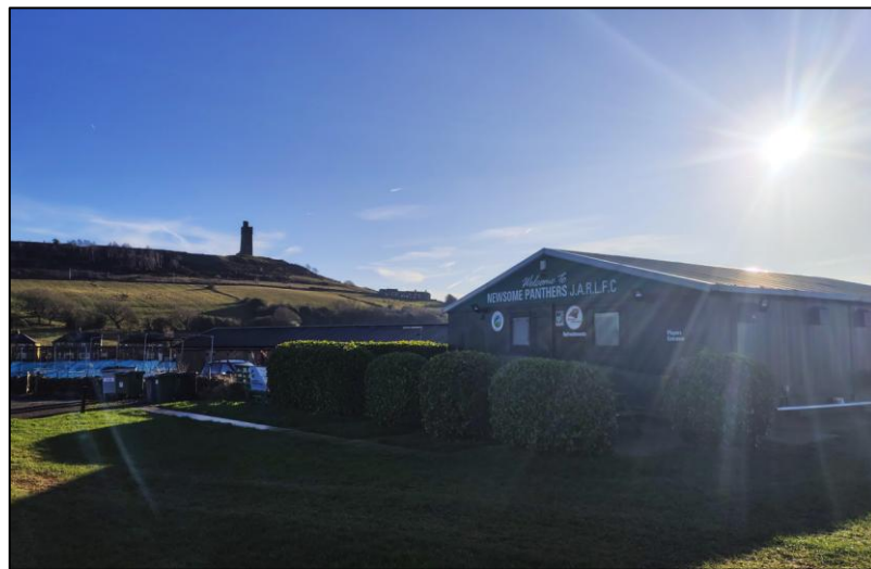
Plate 19. NW gable end of the current Club House with Castle Hill in the far distance
