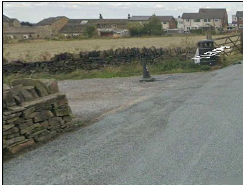
Figure 3 Existing access from the Hall Bower Lane
