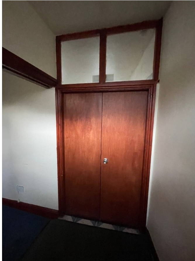
Figure 3: Interior lobby — door leading to the existing body wash room. Plain, utilitarian finishes throughout with no historic fabric present.
