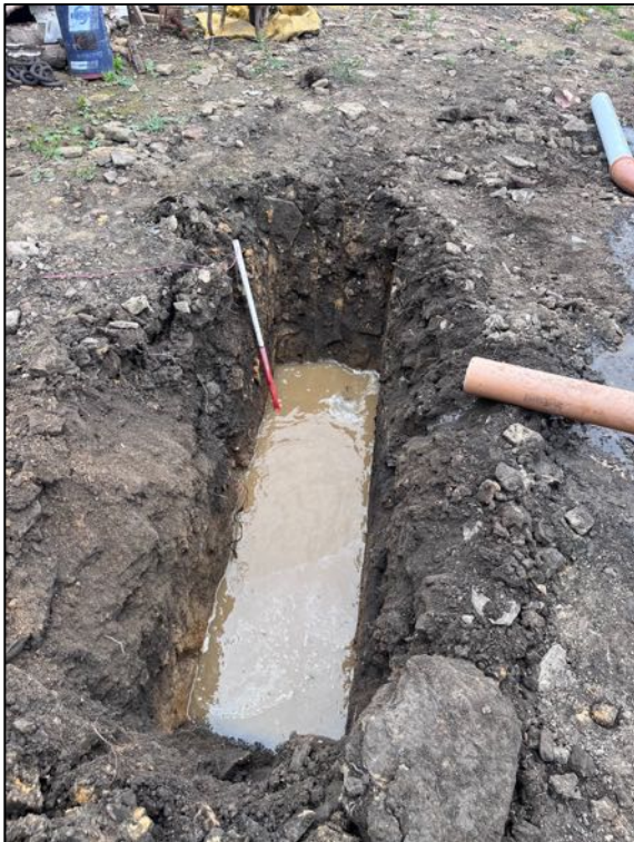
TP4 soakaway test after 1 hr
