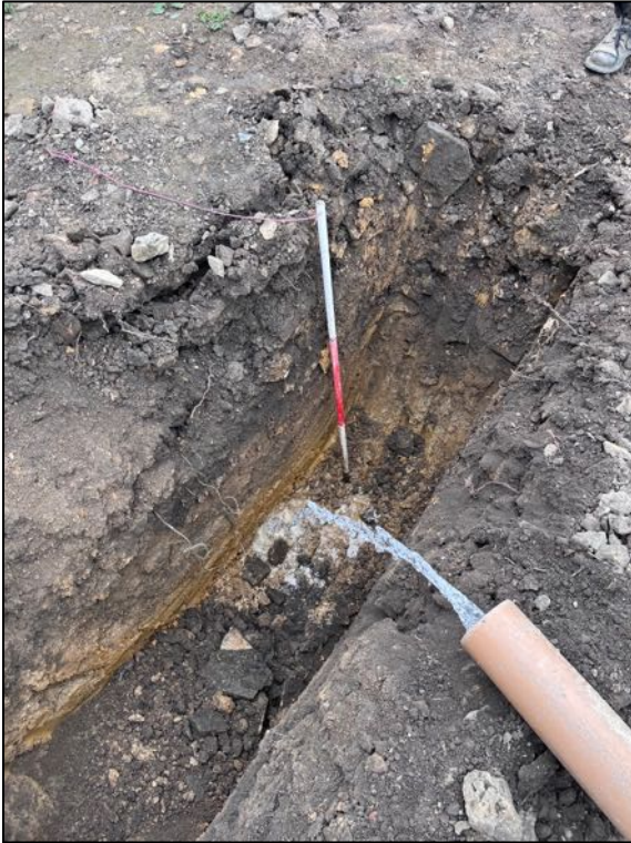
TP4 filling operation for soakaway test
