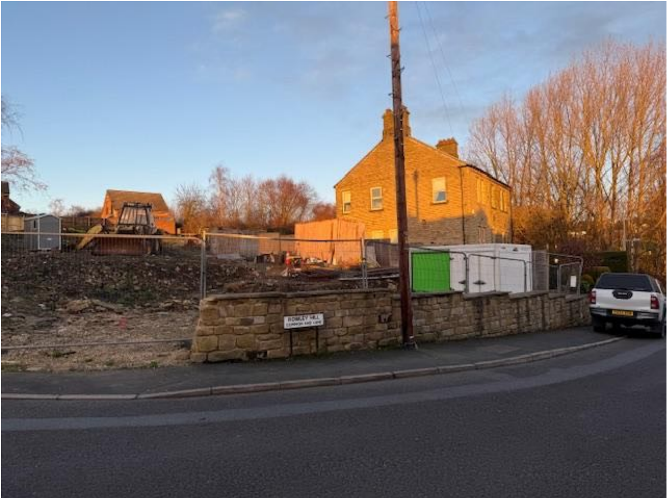
Taken on site.
