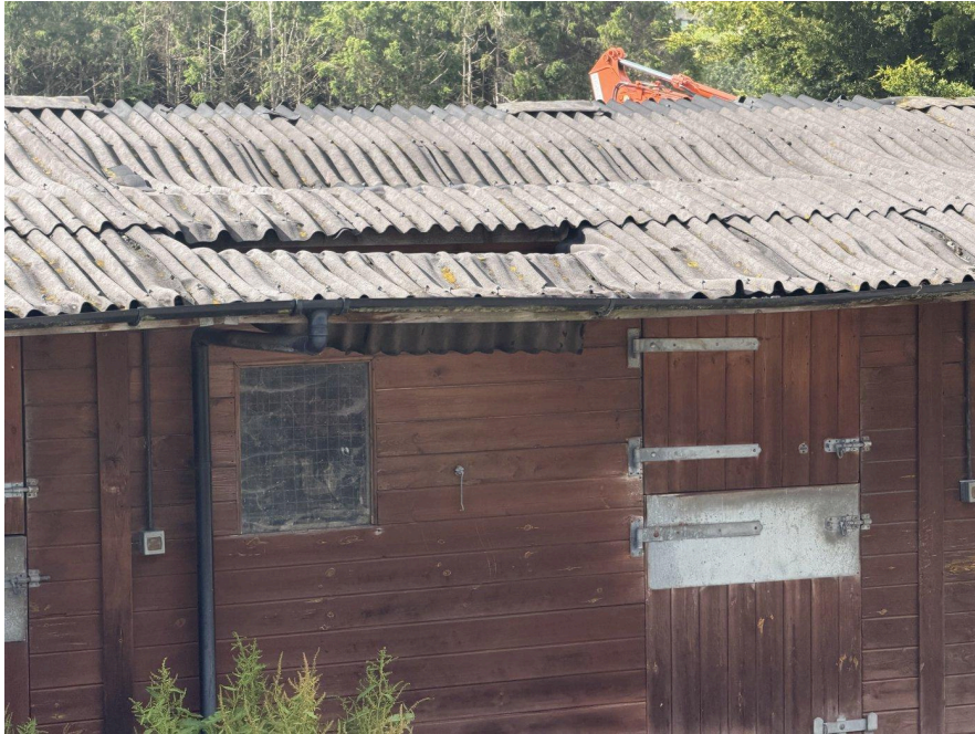
Photograph 1 — External elevation: weathered corrugated fibre-cement roof sheets laid over timber purlins; no enclosed roof void.
