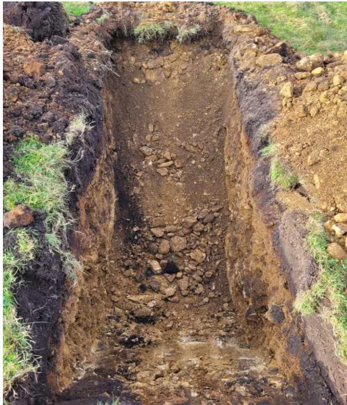
Typical trial pit
