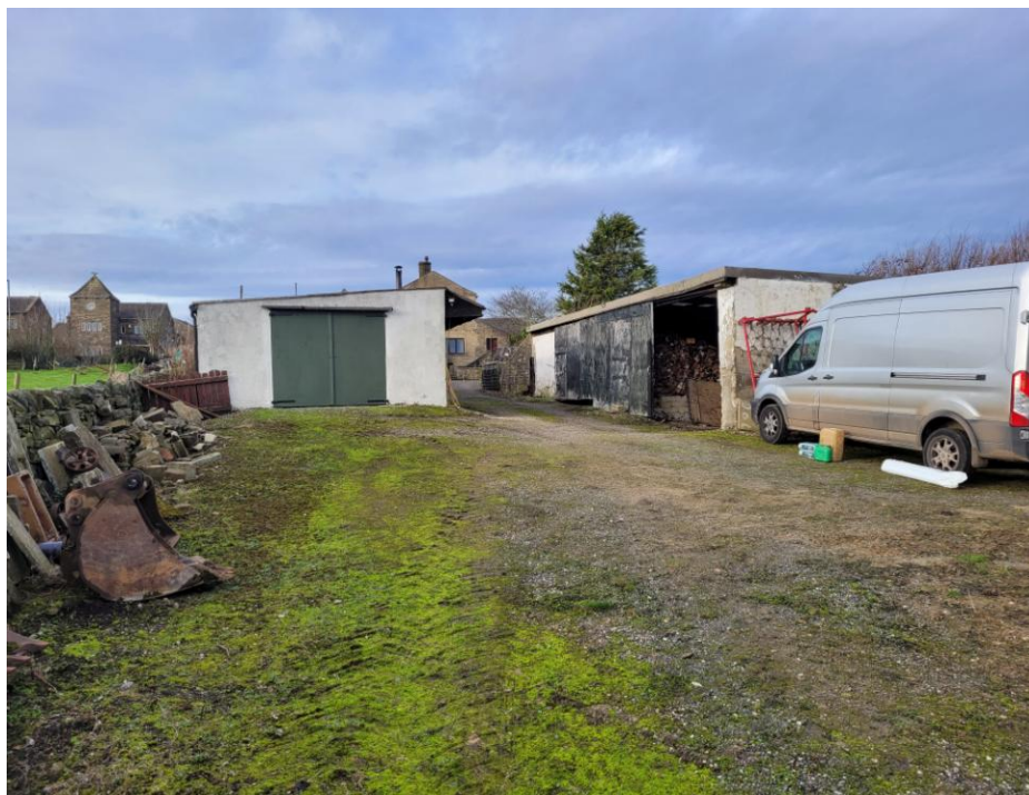
View of stable and barn, looking to the west
