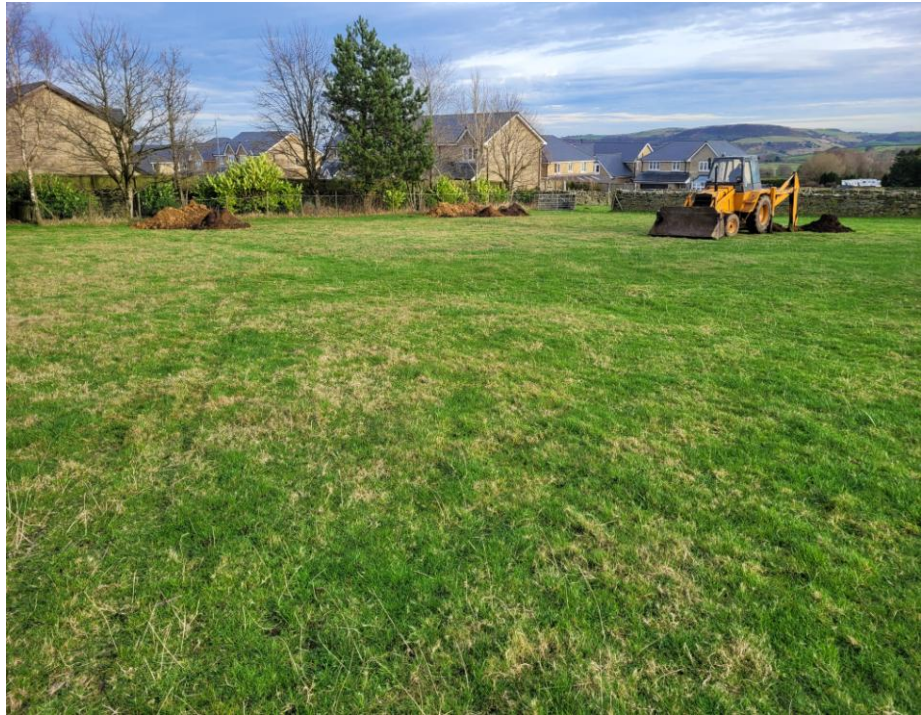
View of western half, looking to the northeast
