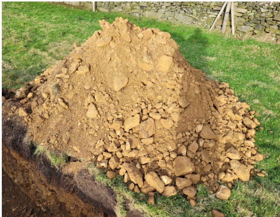
Typical arisings from trial pits
