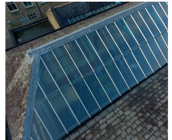
Typical View of Main Roof Glazing Section
