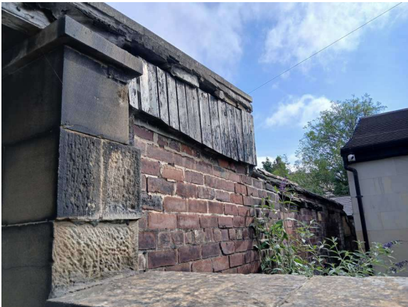
Building B2 – north-eastern elevation
