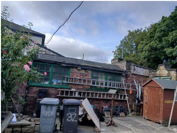
Building B2 -southern elevation
