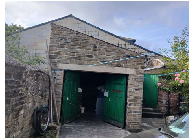
Building B1 – southern elevation
