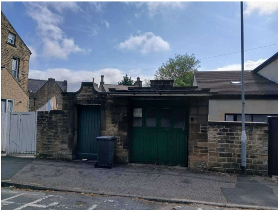
Building B2 – eastern elevation
