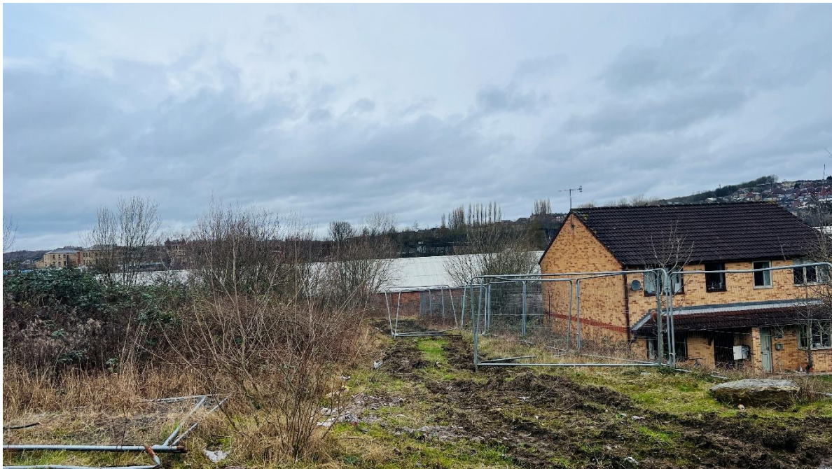
Plate 2 View across the Site, looking north
