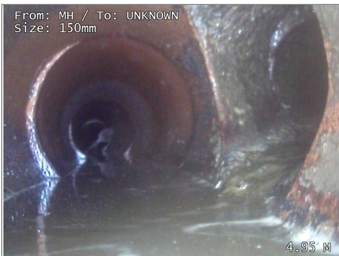
Junction at 3 o'clock, diameter 100mm
