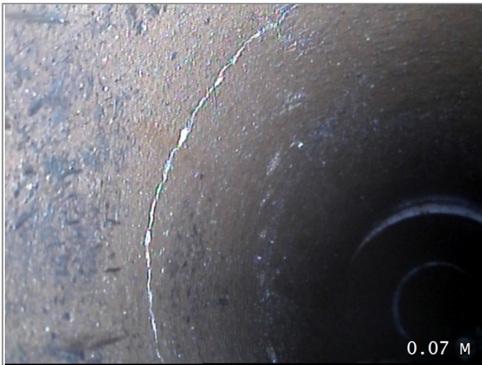
Start node type, manhole, reference MH1
