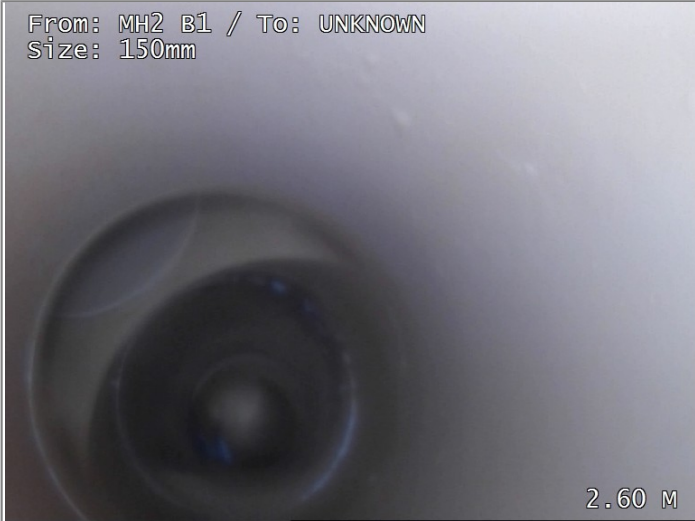
Junction at 9 o'clock, diameter 100mm
