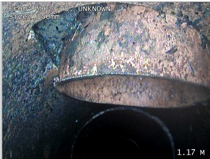
Junction at 12 o'clock, diameter 100mm - Remark: PERTUDING
