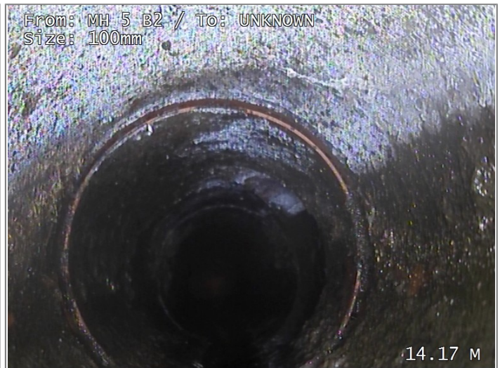
Junction at 5 o'clock, diameter 100mm
