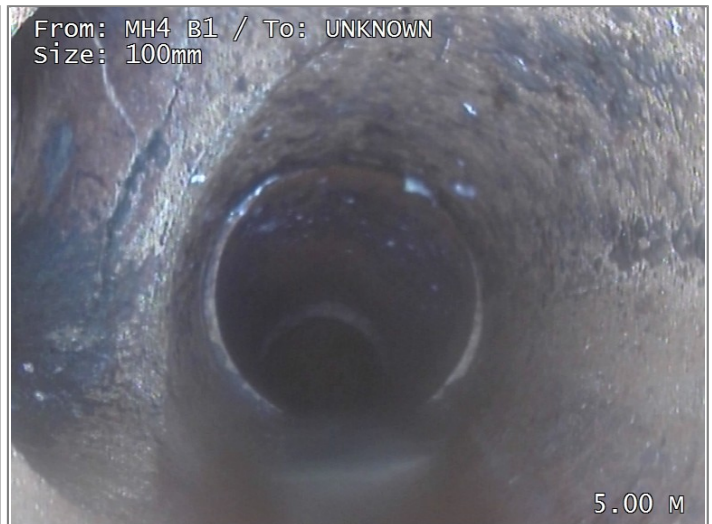
Junction at 9 o'clock, diameter 100mm
