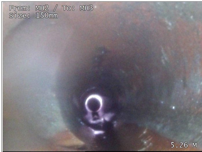
Junction at 9 o'clock, diameter 100mm
