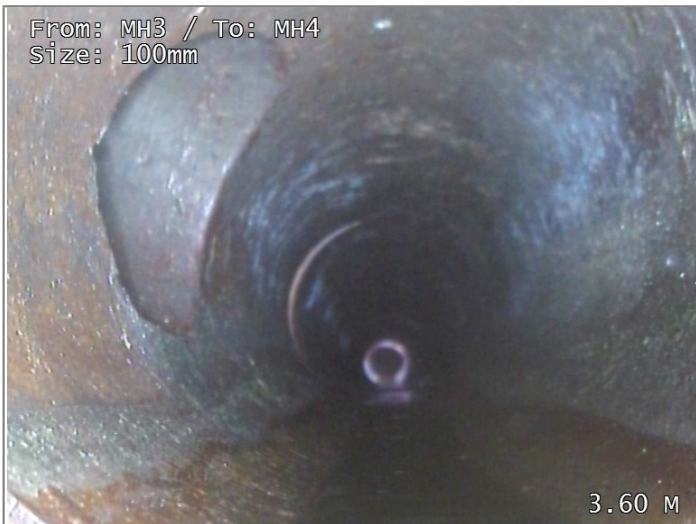
Junction at 10 o'clock, diameter 100mm
