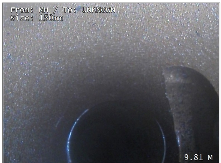
Junction at 3 o'clock, diameter 100mm
