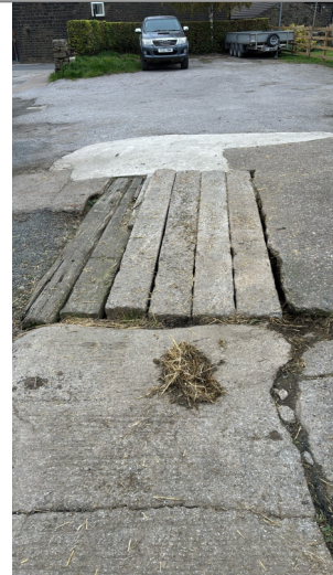
Other Site Photos: Cesspit
