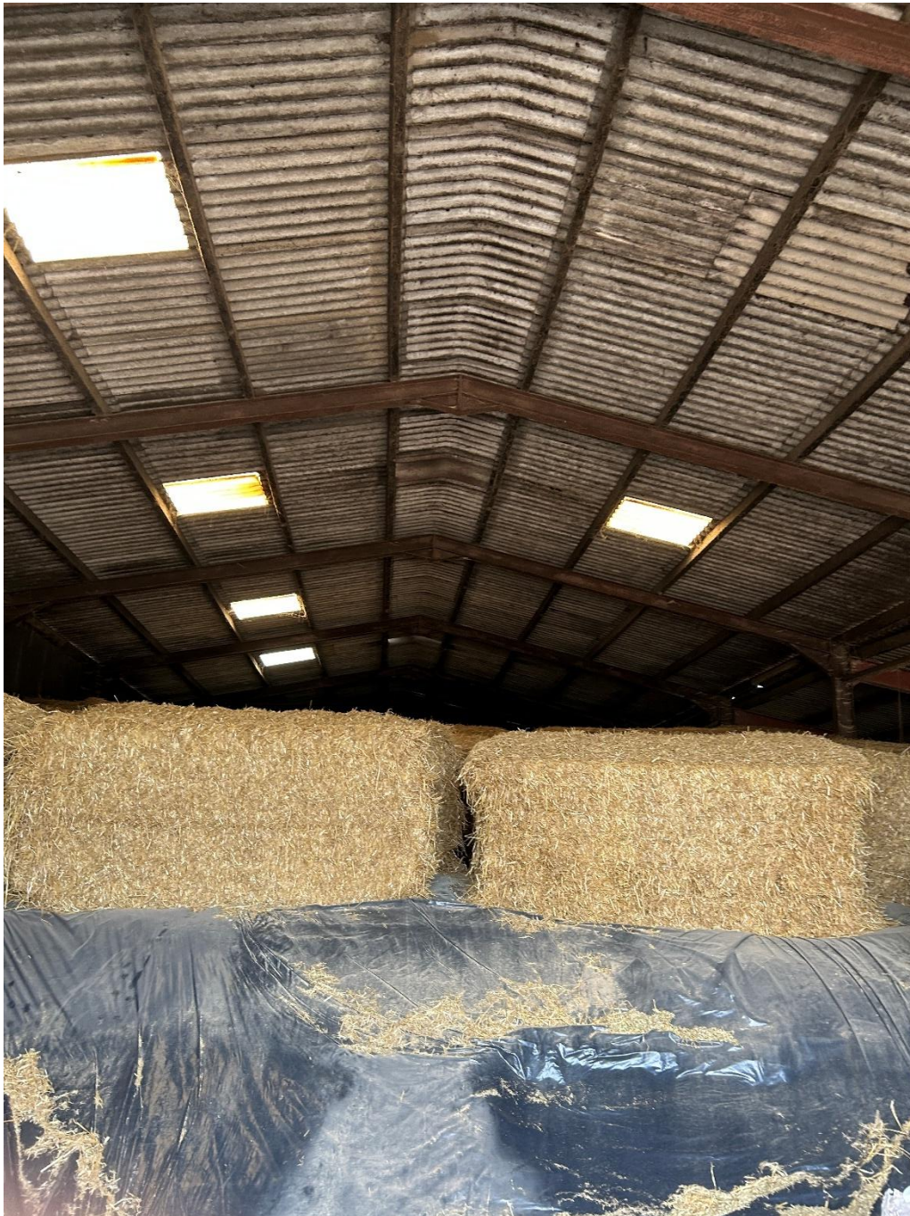
Barn 2 Internal view
