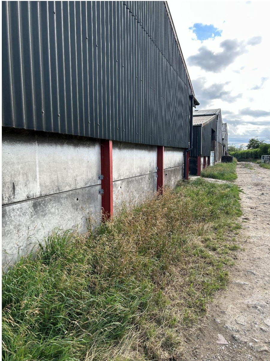
Barn 1 View on gable
