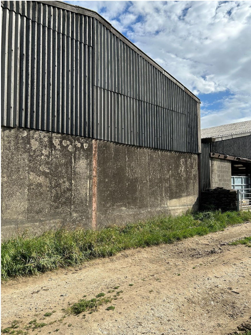
Barn 2 View on gable
