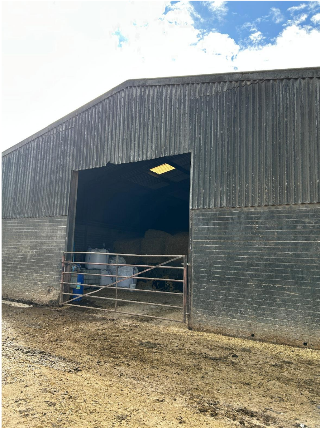
Barn 2 View on gable
