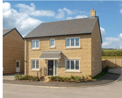
Mix of stone and render façades
