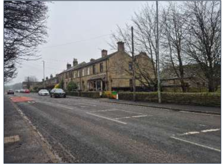
Figure 8 Cottages on south side of Penistone Road, opposite the mill
