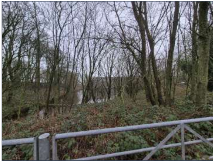
Figure 7 View of the mill from The Bridge with the mill pond in the foreground
