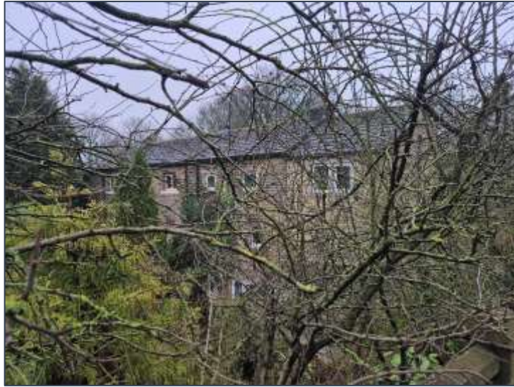
Figure 6 Nos. 1 & 2 The Bridge on approach into Birdsedge
