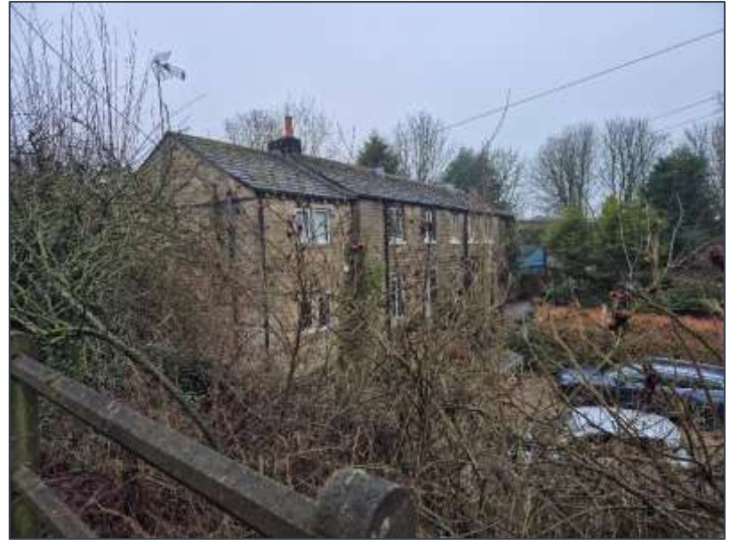
Figure 29 Nos. 1 and 2 The Bridge with two-storey extension on its west
