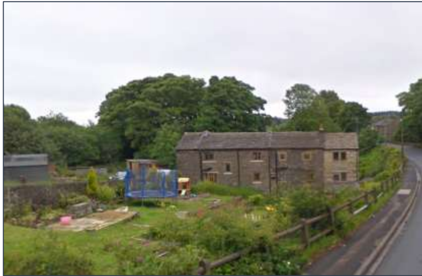
Figure 28 Nos. 1 and 2 The Bridge in 2011 prior to more considerable screening to the roadside. Image from google streetview.
