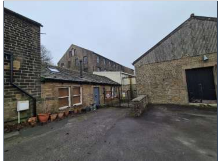
Figure 21 Birdsedge Mill from the south, largely obscured by later C19th additions
