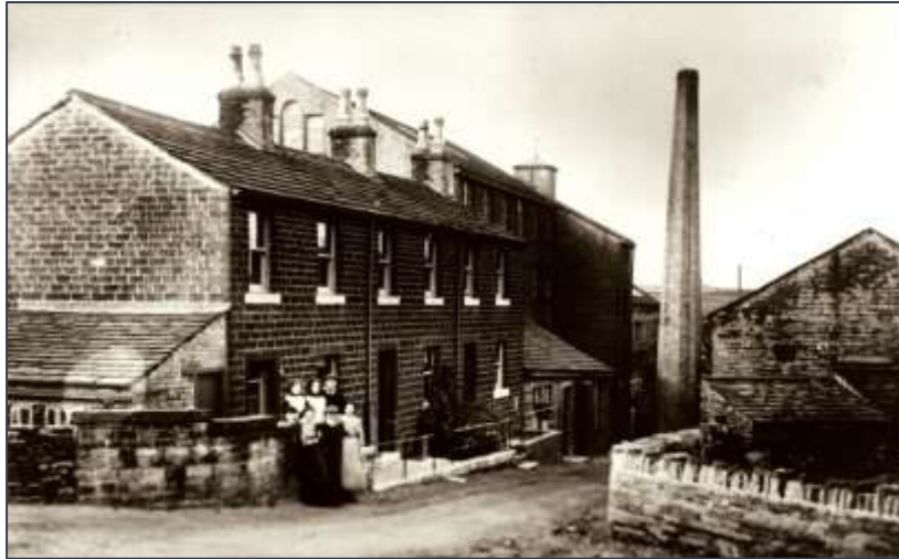
Figure 23 Mill Cottages c.1900
