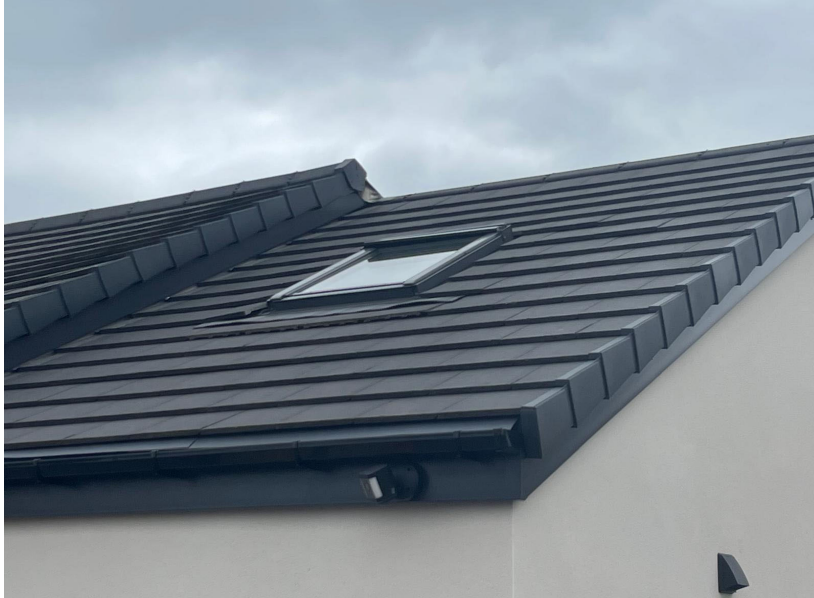
Front Velux window installed
