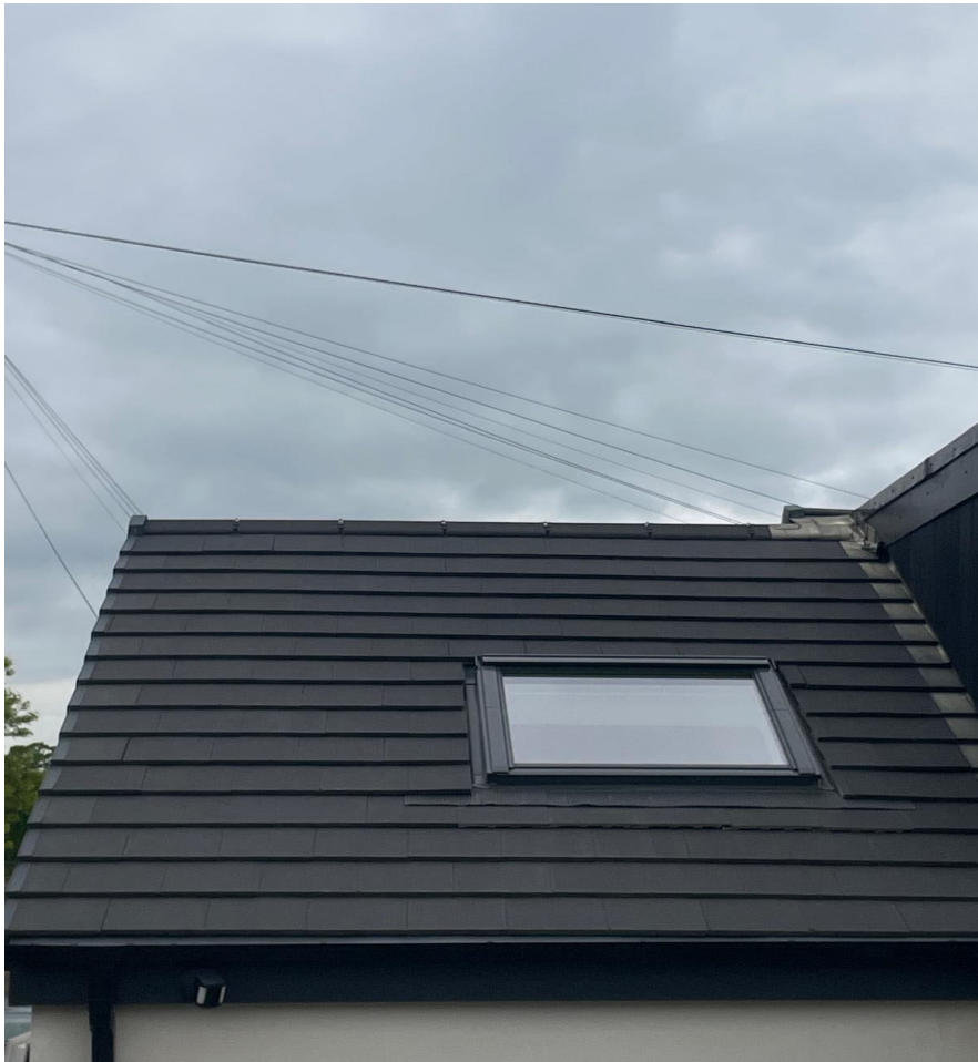
Rear Velux Window installed
