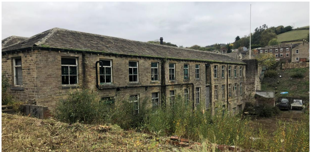
Photo 1. Hinchliffe Mill from the south east
