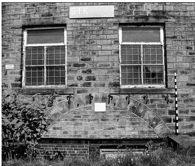
Photo. 2. Arch at north end of west elevation
