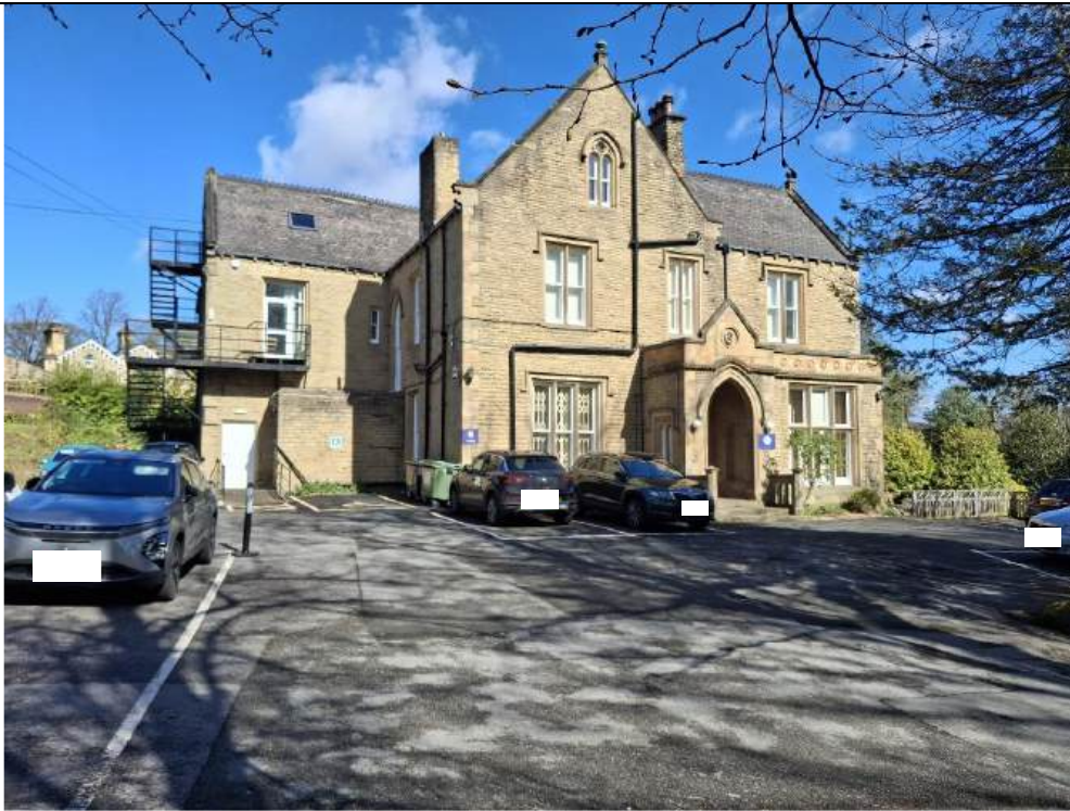
Photo 3: Main building. Taken at southwest corner of site looking north.
