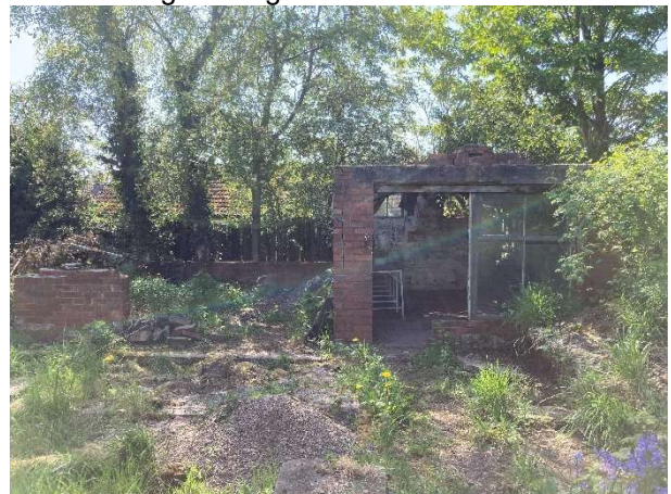
Photo 6: Building 1 on the southwest of the site.
