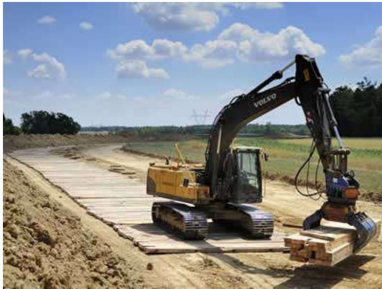
Figure 1: Example bog mats (© Briketts https://www.birkettsbogmats.com/size-bogmat/ )
