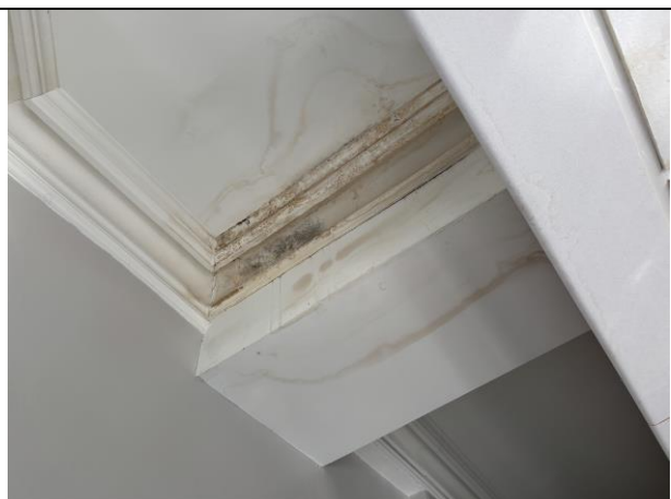
Photo 6 – Internal leak
