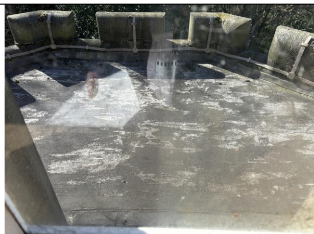
Photo 5 – Asphalt deterioration
