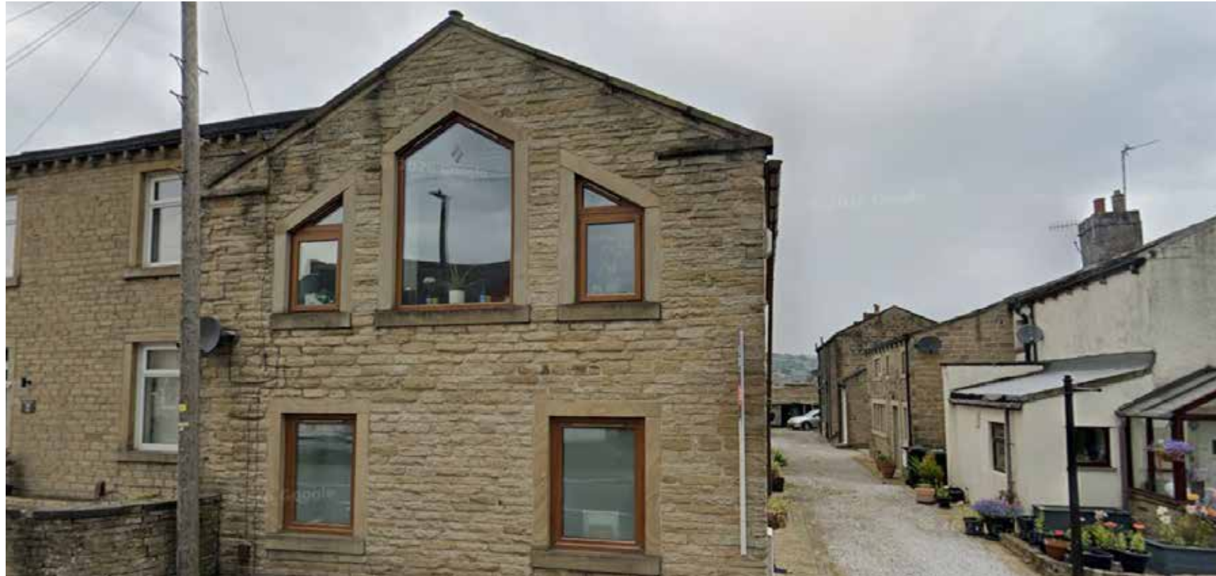
56 A Hazel Grove as seen from the front of Hazel Grove
