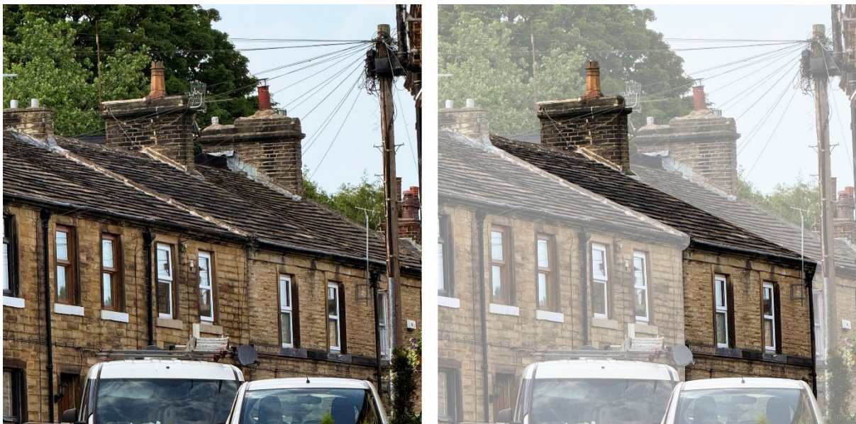
Figure 2 – Existing roof slope showing natural stone slate roof covering.
