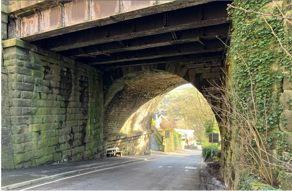
Figure 10: North entrance from Bank Gate, showing the later viaduct in front of the original arch.
