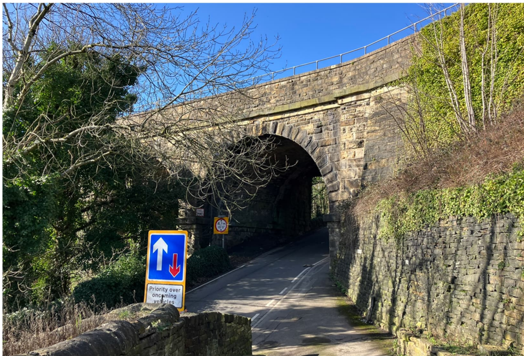
Figure 9: South elevation of Slaithwaite Viaduct, with Bank Gate, from Ivy Mount road.
