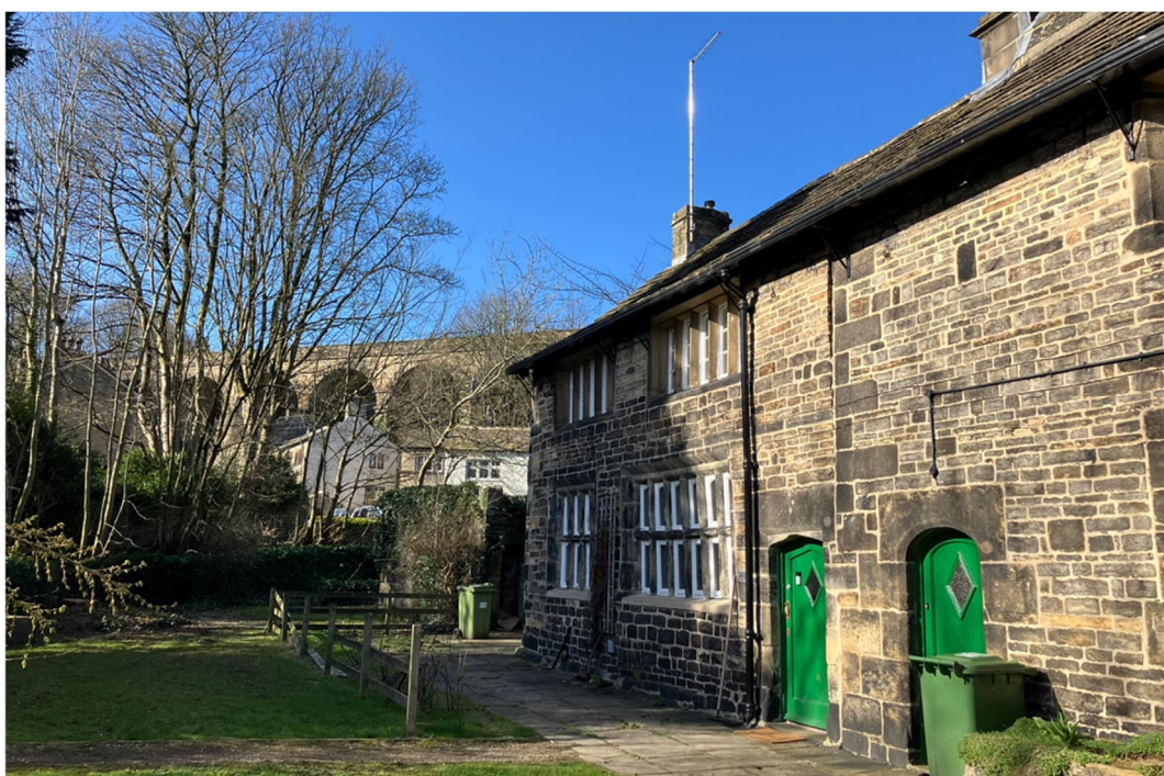
Figure 16: Looking north west to the viaduct from the Manor House.
