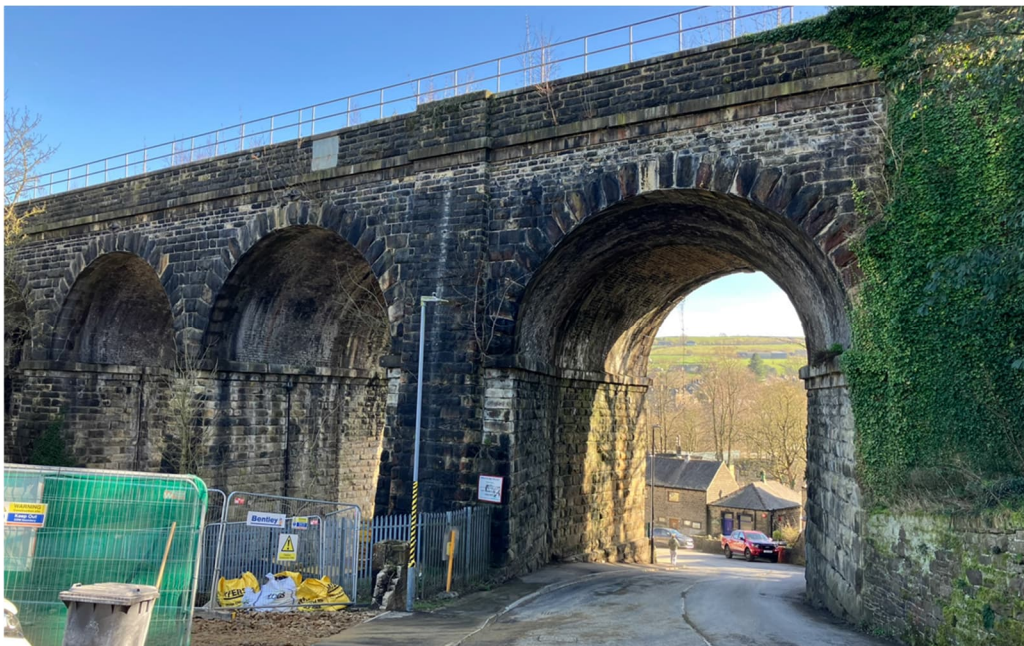
Figure 11: North elevation of viaduct from Nabbs Lane, looking south into conservation area.
