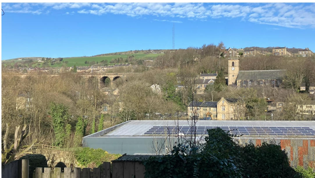
Figure 14: Glimpsed views of the viaduct looking north from the A62 Manchester Road.
