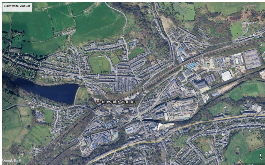
Figure 8: Slaithwaite Viaduct, 2026. Copyright Google Earth under Creative Commons licence.
