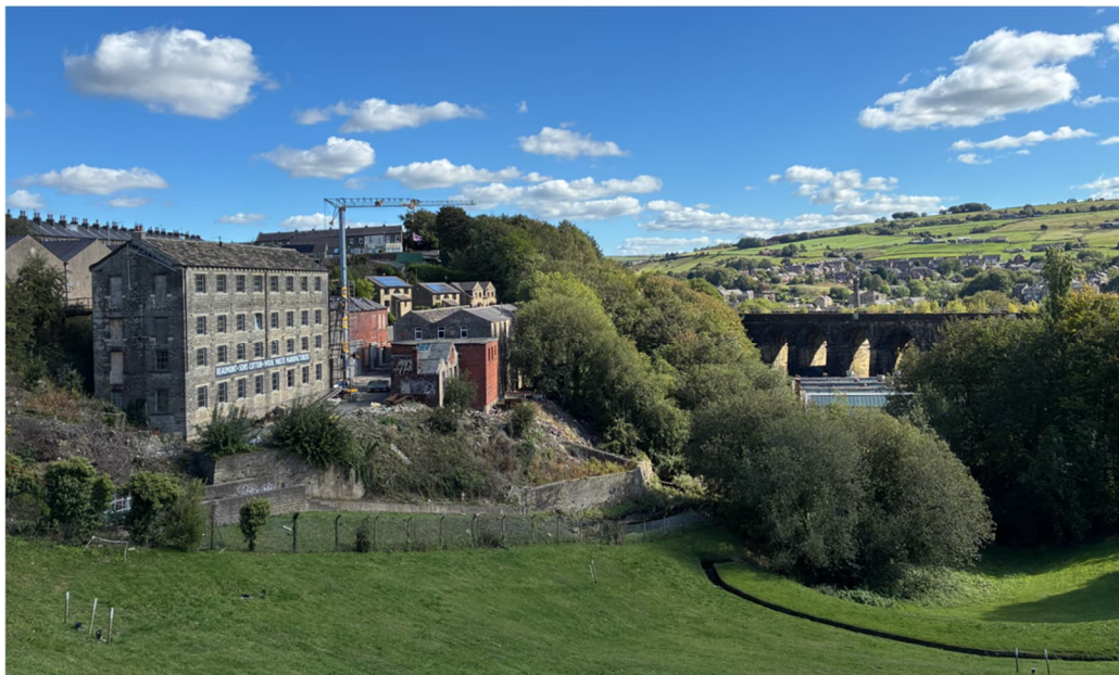
Figure 12: North elevation of Slaithwaite Viaduct and Bank Gate Mill, looking south east from Slaithwaite Reservoir dam.
