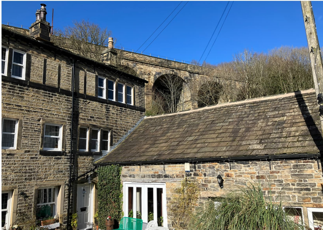
Figure 17: Looking north east to the viaduct from listed 11 Nabbs Lane.
