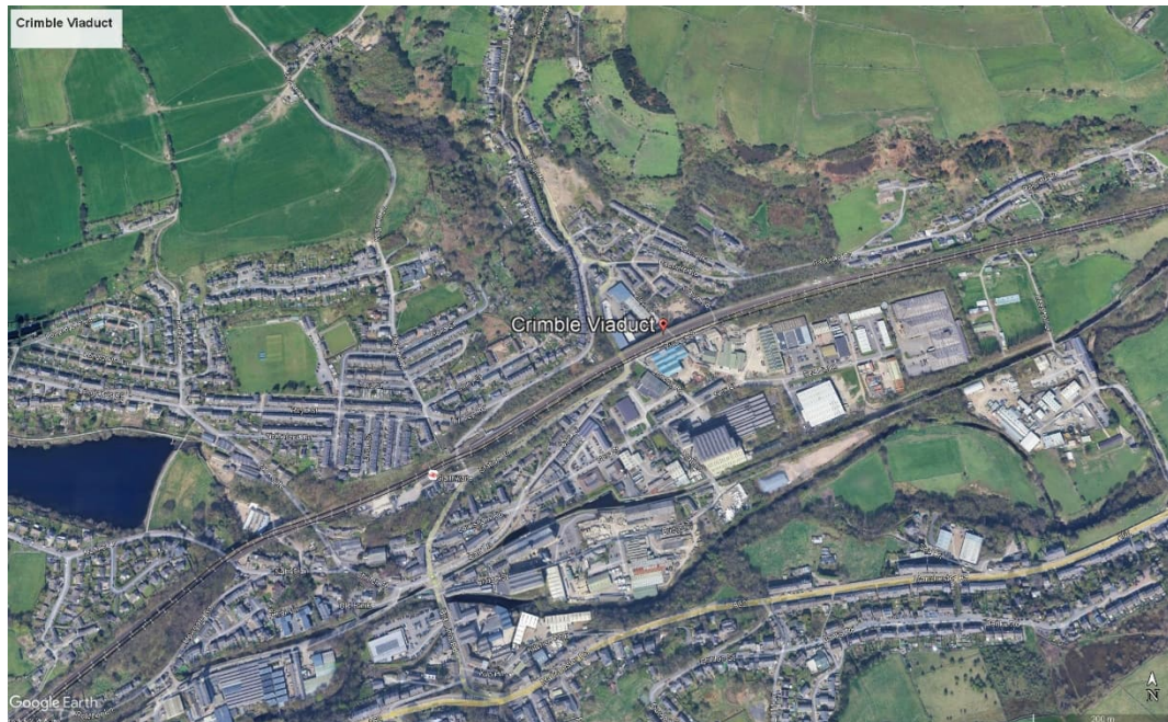
Figure 8: Crimble Viaduct, 2026. Map Data © 2026 Google, Airbus.
