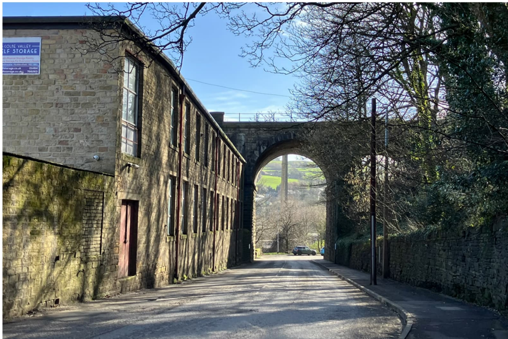
Figure 13: Looking south down Carr Lane to listed Platts Mill Chimney.
