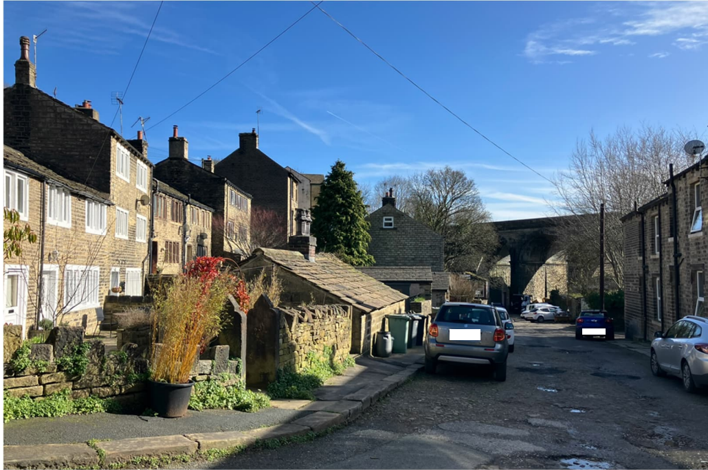
Figure 12: Looking south down Knowle Road, listed weavers' cottages to left, north elevation of viaduct to right.
