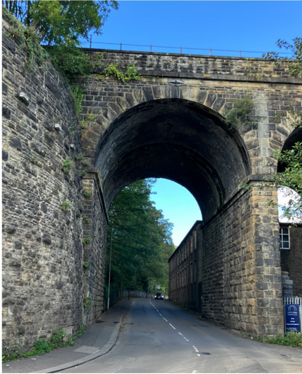
Figure 10: Crimble Viaduct, looking north from Carr Lane.
