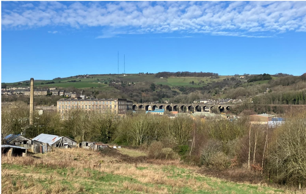
Figure 11: View of Crimble viaduct looking north from A62 Manchester Road with five storied part of Spa Mill in the foreground, adjacent to the listed Platts Mill Chimney.
