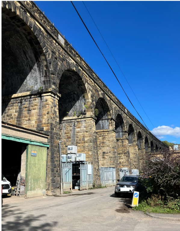
Figure 9: Crimble Viaduct looking east from Carr Lane.
