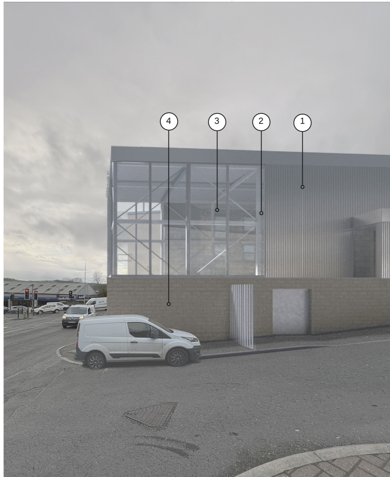
Corrugated metal cladding
