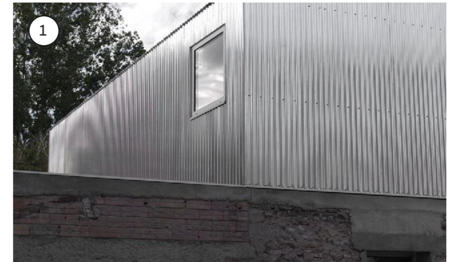
Corrugated metal cladding
