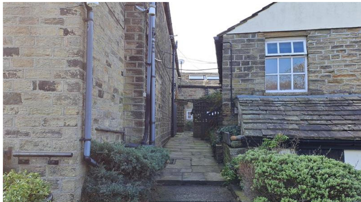
Photo 17: View of passage between the existing residential properties and the ancillary residential buildings - Photo taken from east of centre of site looking west
