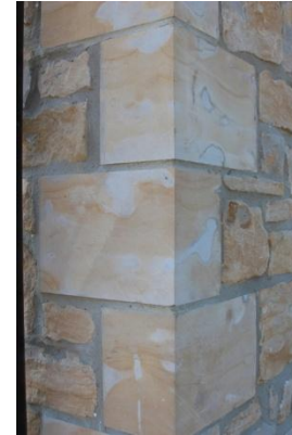
Ashlar stone quoins
