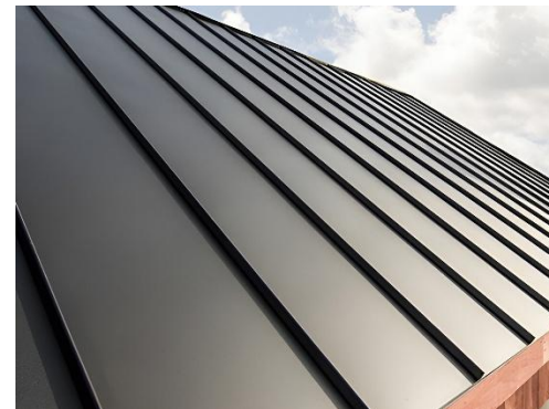
Metal standing seam to Plot 3 extension
