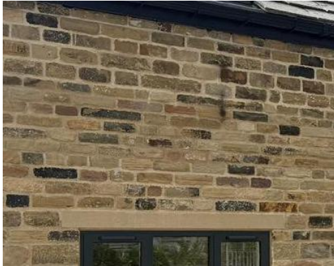
Reclaimed coursed walling stone
