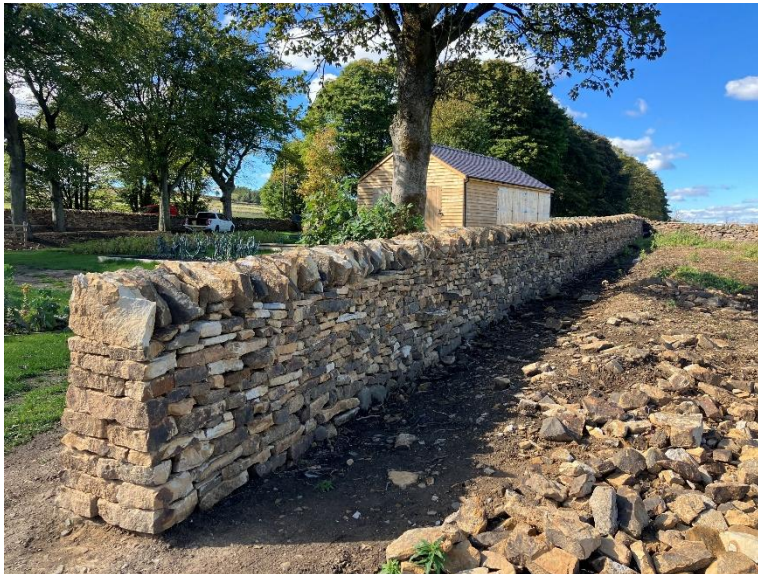
Drystone walls where walls are shown on site layout. Max 1.2m high
