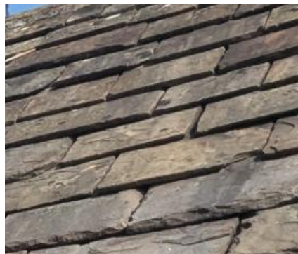
Reuse stone slates from stables and out buildings or source similar
