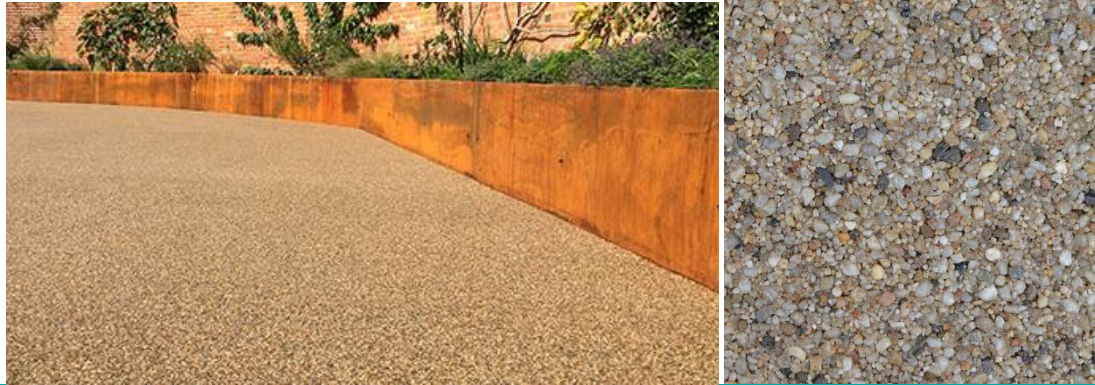
Resin bound gravel drives and access tracks
