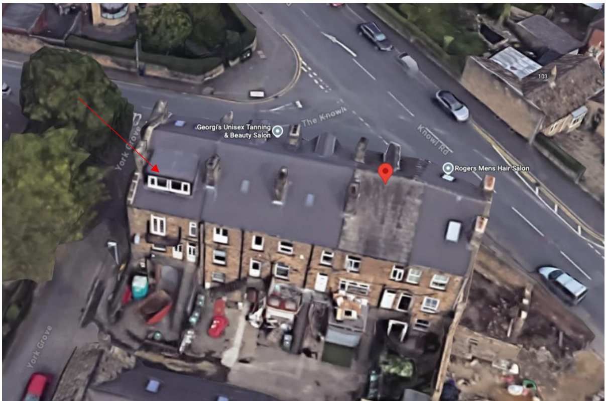
Above: The dormer to the rear of No.7 The Knowl can be viewed along this terrace.
