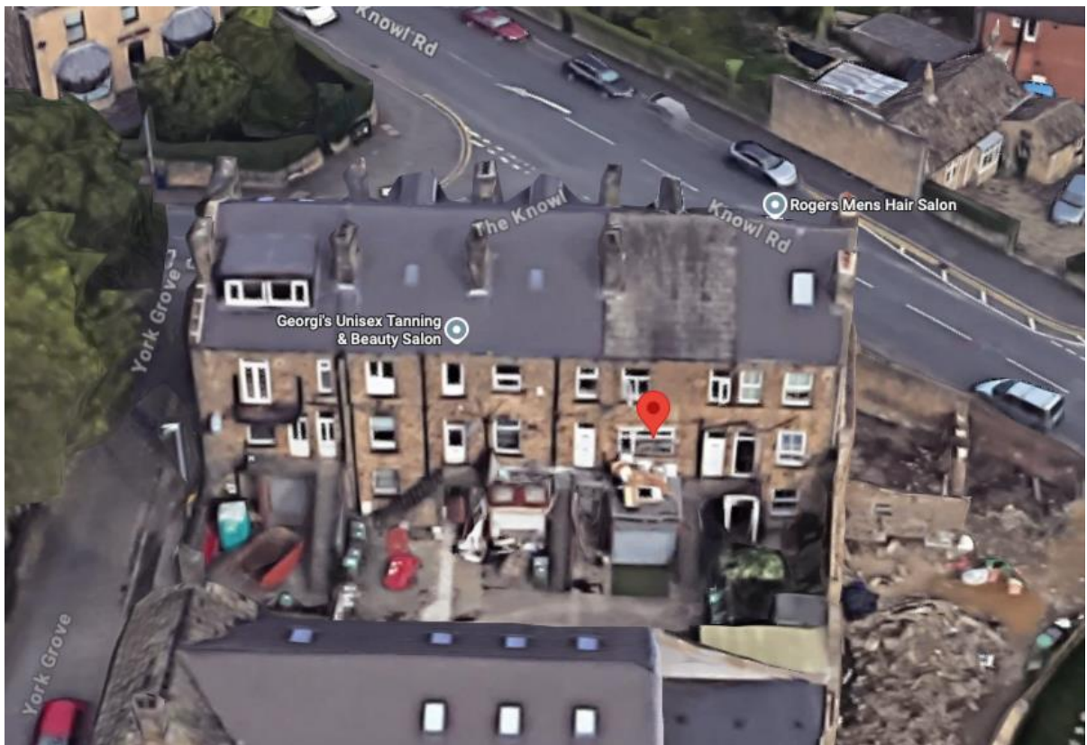
Above: This shows the rear three storey elevation of the property
