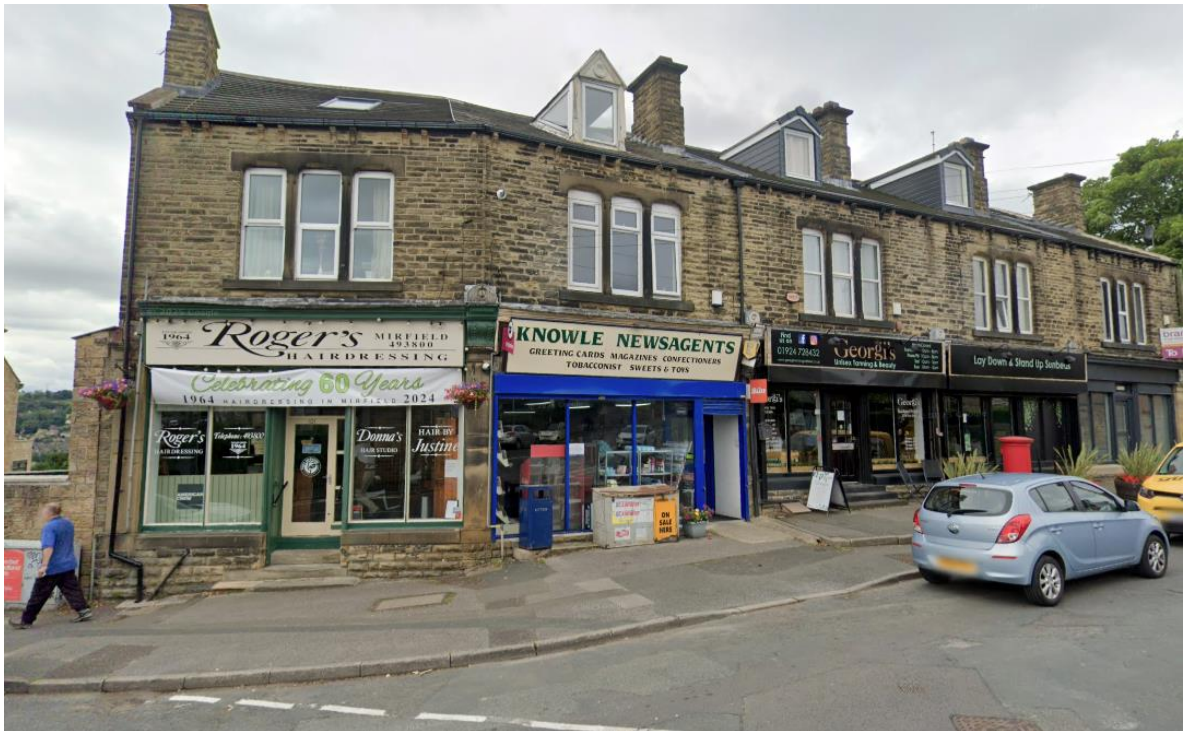
Above: Front elevation of the property with retail at ground floor, upper floors are vacant.
