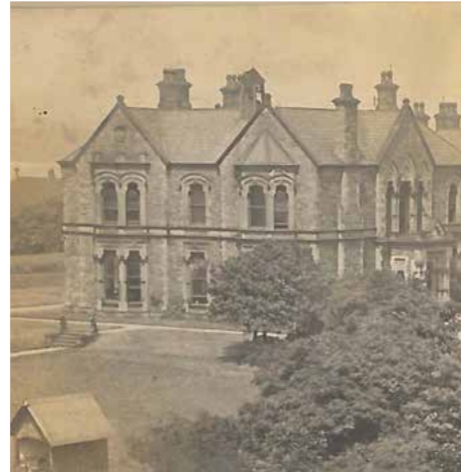
View of the original bay windows
