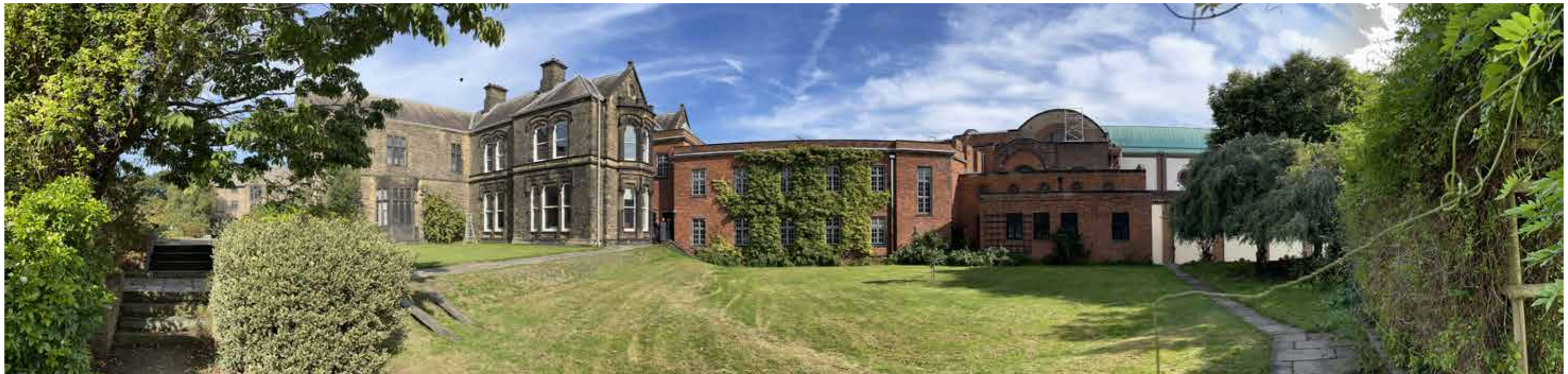
View from the west of the main house and library
