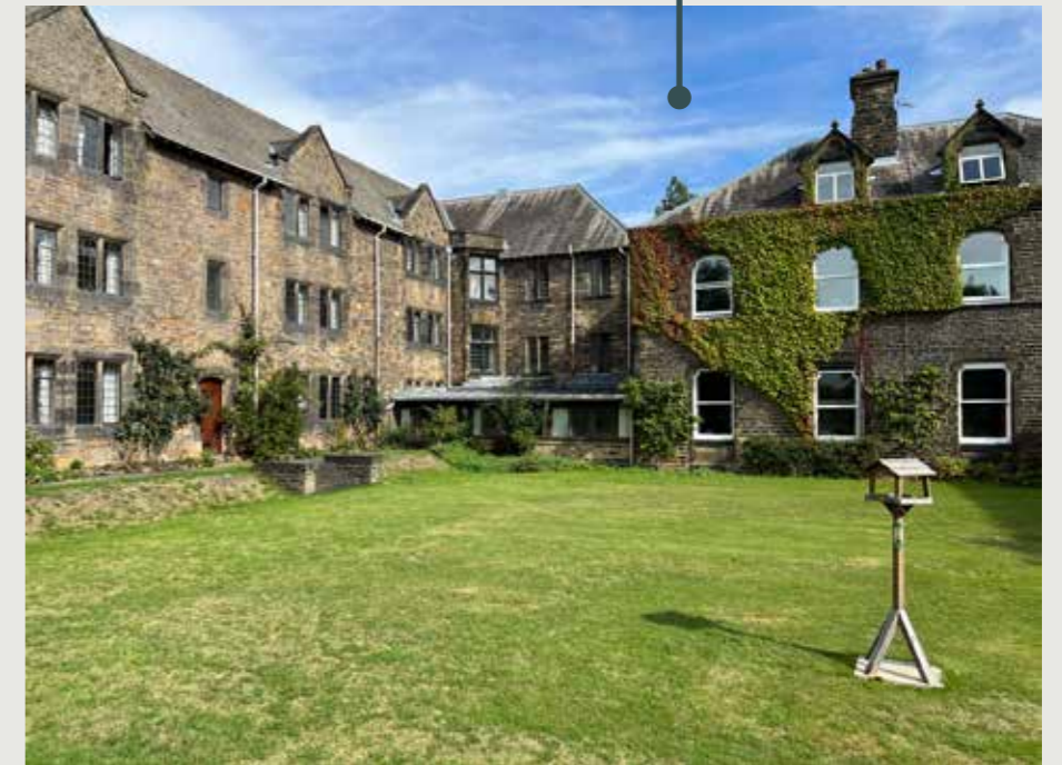
2022 - Showing the infill extension to the rear elevation
