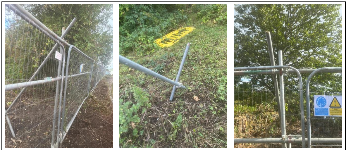
Figure A3.2: Examples of scaffold framework temporary tree protection fencing.
