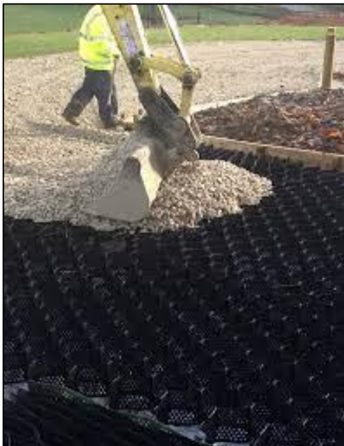
Figure A3.5: Cellweb® geo-cellular confinement sheets being installed.
