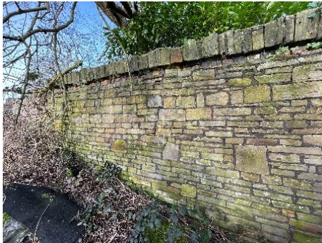
View of retaining wall with negligible bat roost potential.
